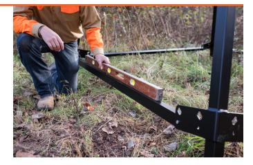
Hook each included cable brace onto the tabs as shown here.
