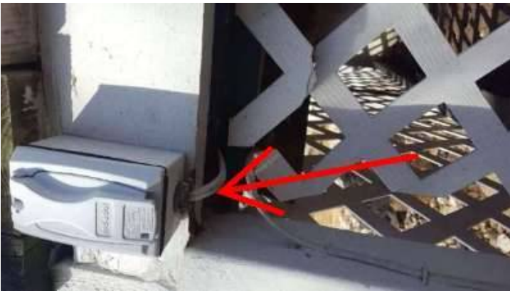
Photo 12-1 All exterior outlets non GFCI. Some have exposed wiring.
