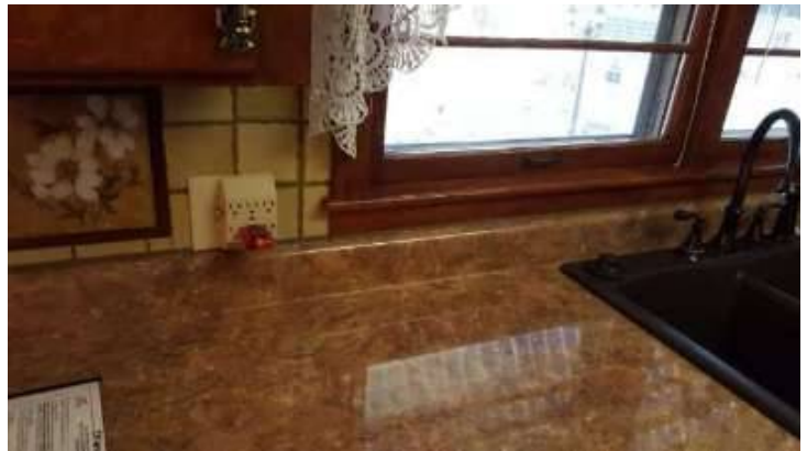
Photo 12-2 All kitchen outlets including Garbage disposal to be GFCI
