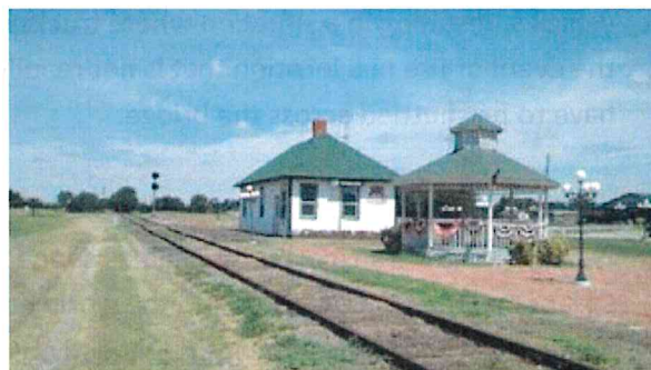
Former Holdenville depot on the discontinued UP line
