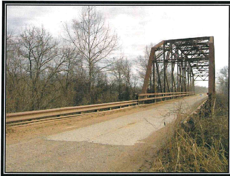
Bridge over the Little River, Hughes County
