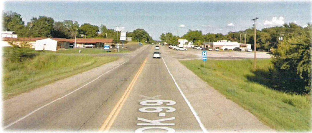
View travelling East on OK 99/64, on the west side of Cleveland. Functional shoulders permit bicyclists or pedestrians to travel off the vehicle lanes of the road to access businesses such as a mini-storage facility, budget motel and restaurant. The shoulders end about a mile west of town. No Bike/Ped signage or rumble strips are present.
