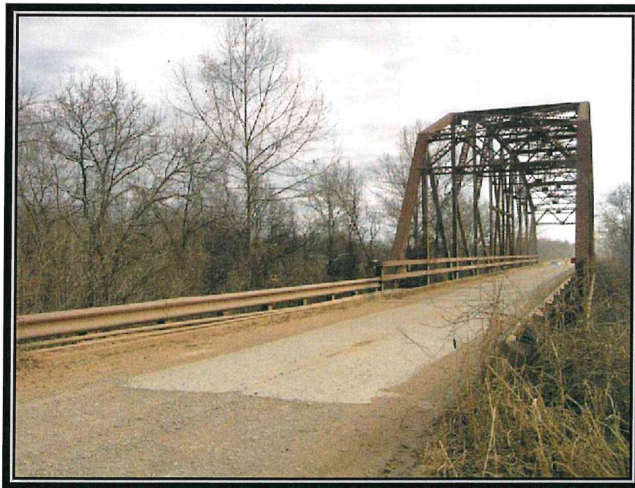
Bridge over the Little River, Hughes County
