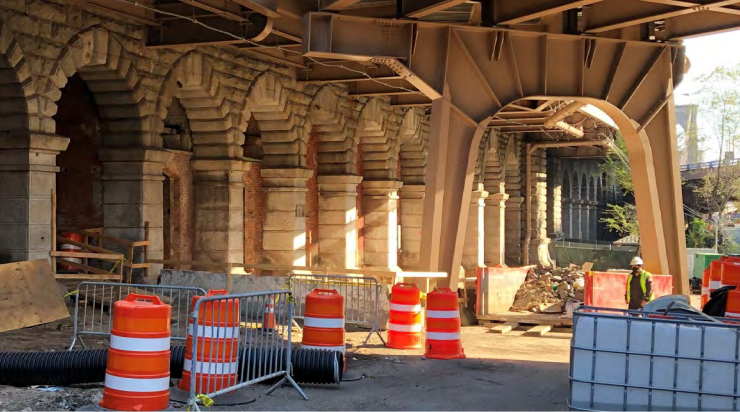
STAGING AND STORAGE
