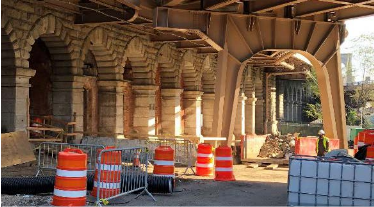
STAGING AND STORAGE
