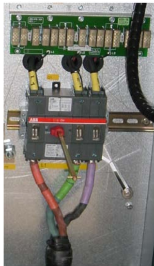
Input Cable Connections Figure 2.
