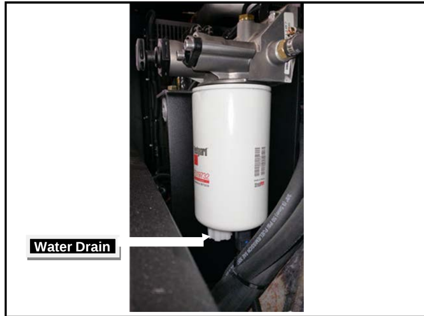
Figure 2-1-2 Fuel Lubricity Drain
