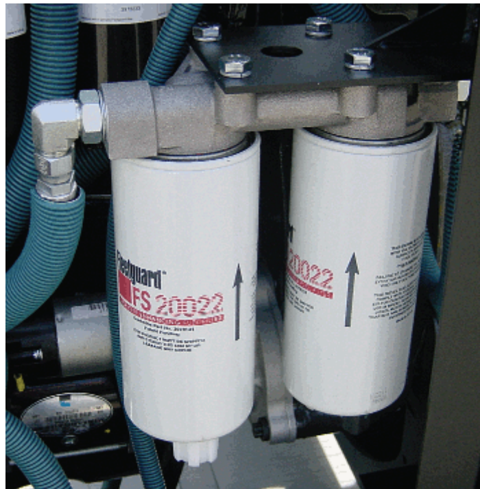
Lubricity Filter Element (286897-031)
