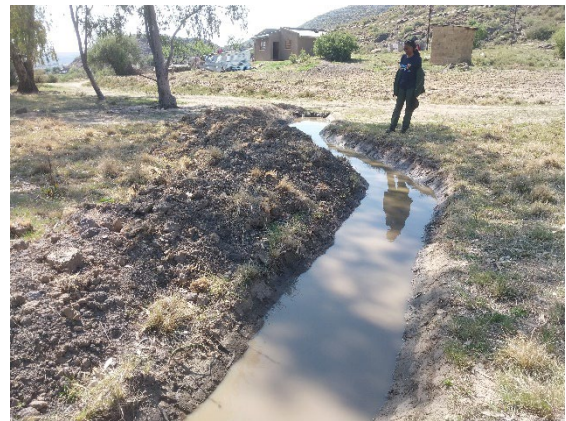
Fig. 13: winter rain halted by a new swale Lithakaling Primary School.
