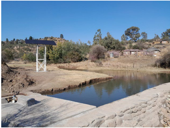
Fig. 2: Sand dam and solar pump Waterfall Village.
