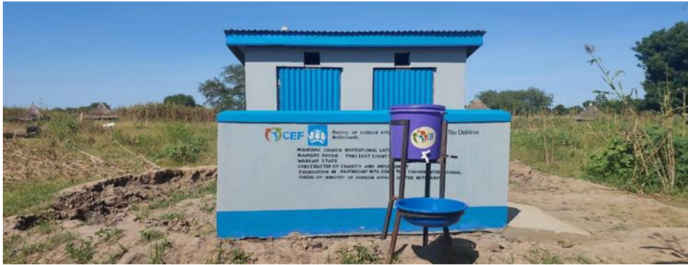
Figure 12: Institutional latrines with hand washing facilities in Palal Payam, Tonj East County 2023
