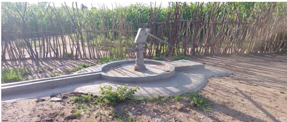
Figure 13: A boreholes rehabilitated in Makuach Payam in Tonj East County, 28/9/2023
