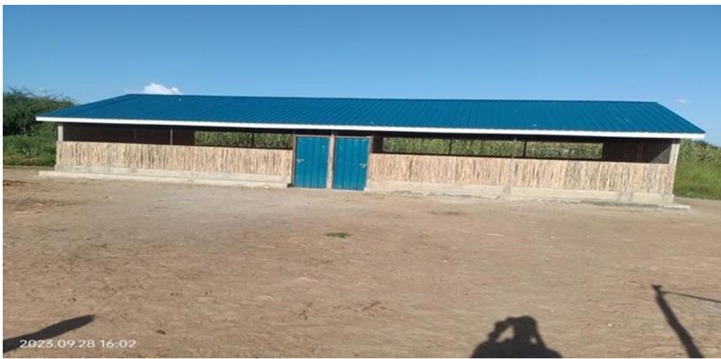
Figure 8: TLS constructed with the UNICEF Funding in Awerial County, 2023
