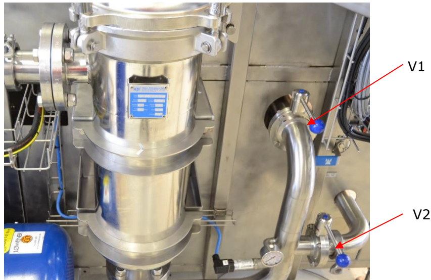
Fig. 5.8 Valve settings tank flush wash
