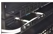
70mm panel for cable management
