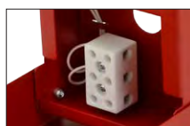
Porcelain screw connection in cabinet
