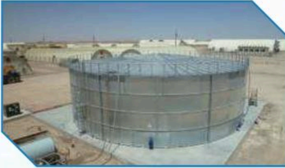
Kandahar / Şantiye Su Deposu (AFGANİSTAN) - 855 ton Kandahar / Site Water Tank (AFGHANISTAN) - 855 ton
