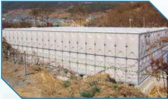
Kazakistan / Arıtma Tesisi - 880 ton Kazakhstan / Treatment Plant - 880 ton
