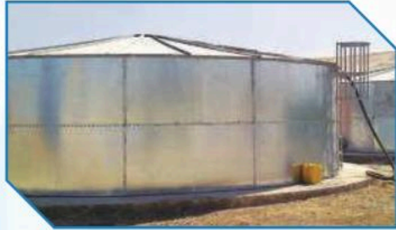
Kandahar Amerikan Üssü Su Deposu (AFGANİSTAN) - 150 ton Kandahar American Base Water Tank (Afghanistan) - 150 ton
