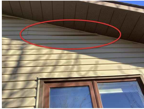
Re-install Siding
