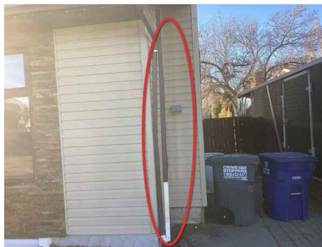
Relocate or extend downspout
