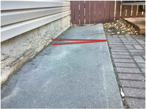
Sidewalk has Sunken
