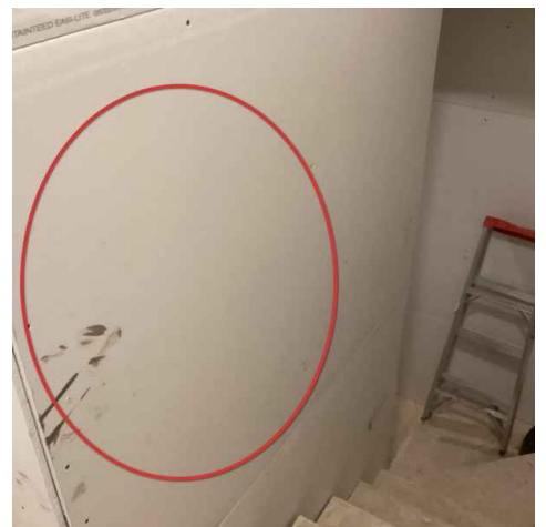
Lack of Drywall Screws
