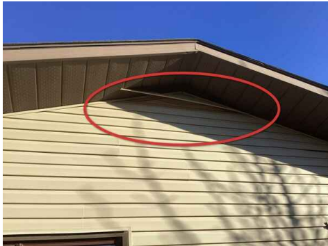
Reinstall Siding
