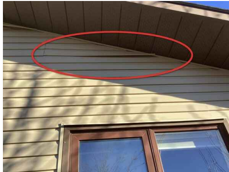
Re-install Siding
