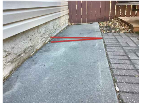
Sidewalk has Sunken
