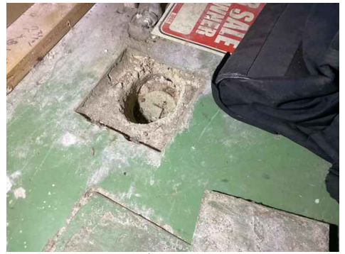
Cast Iron Cleanout to Street
