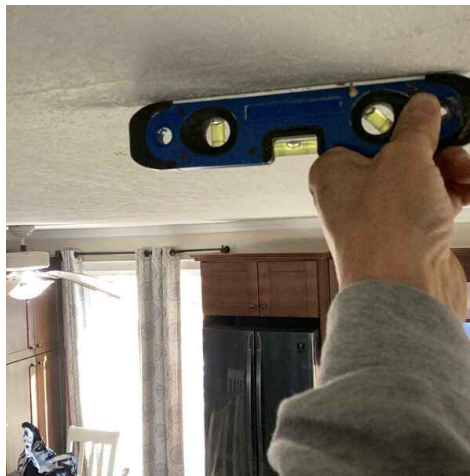
Ceiling is level adjacent to area of concern
