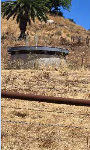
Large pipelines may stretch for miles underground mostly undetected. Here an air relief valve structure reveals the pipeline beneath.
