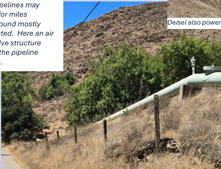
This pipeline runs exposed along the ground feeding a nearby water treatment plant.
