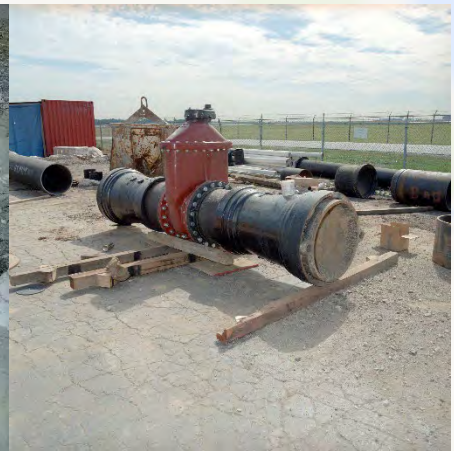
A Large Main Valve Awaiting Installation
