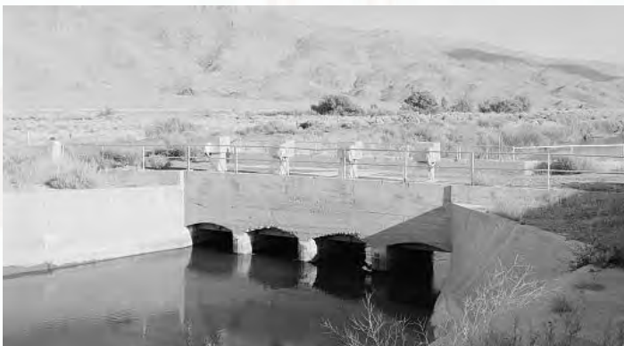
The original water intake to the L.A. Aqueduct
