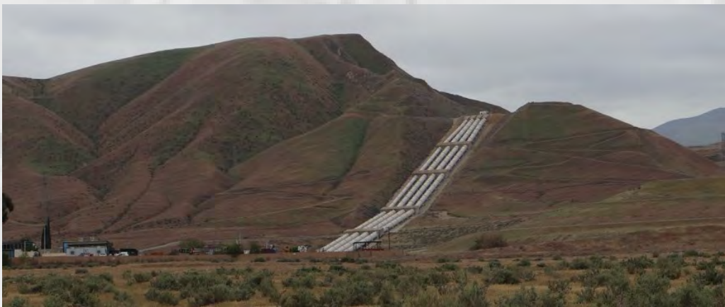
Ira J. Chrisman Pumping Plant, Grapevine CA
