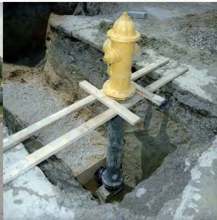
Hydrant Under Construction
