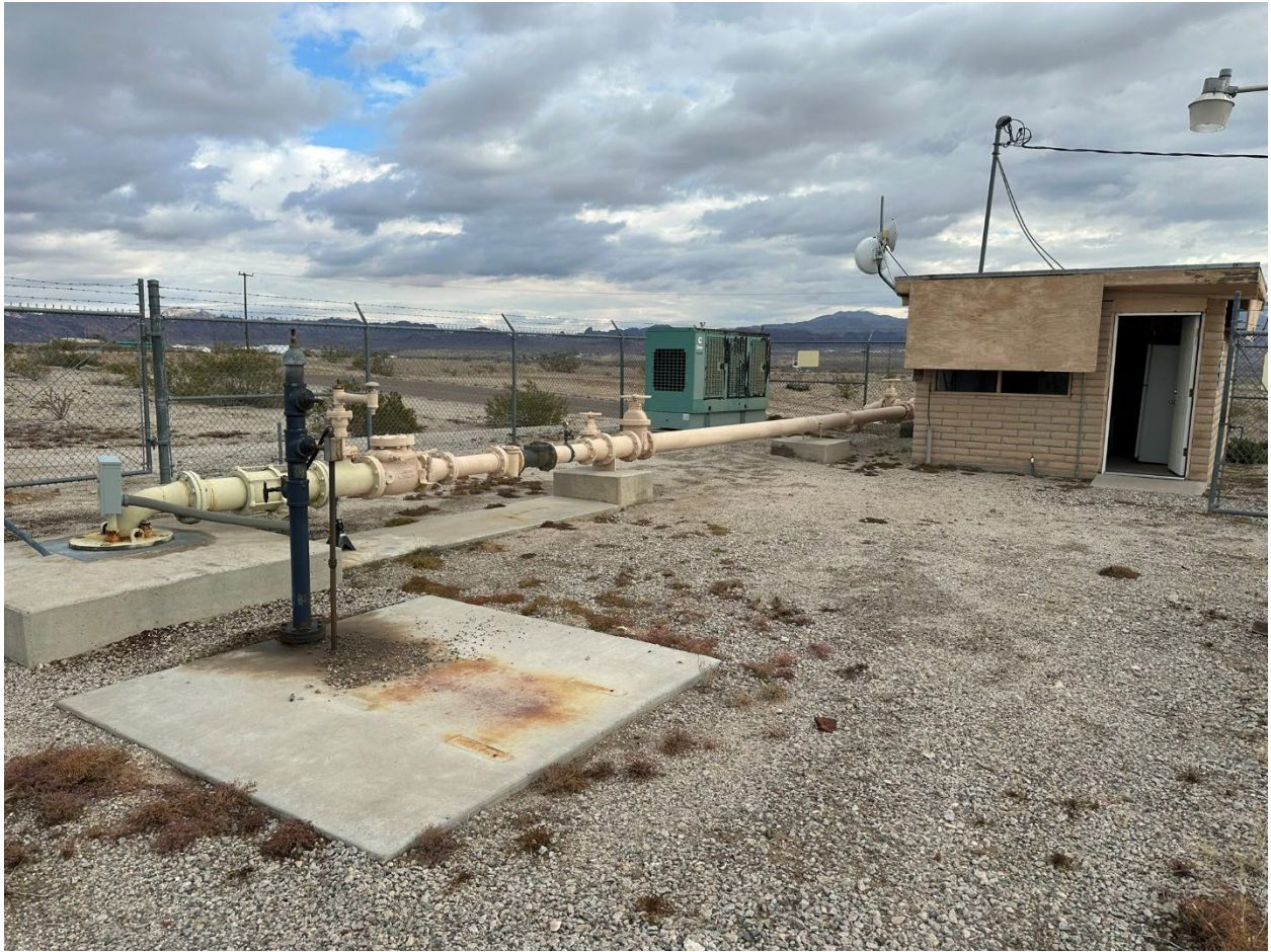
Figure 16: Northeast View - West Well Site
