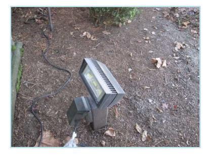
Monument lights are newer LED's and appear to be deteriorating at a rate typical of their age. We recommend budgeting for replacement at the timeframe indicated due to constant exposure to the elements and deterioration of the component over time.
