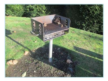
Metal cooking grill is in fair condition. Some surface rust noted. Plan for eventual replacement as these structures will deteriorate from the heat as well as the exposure to the elements.
