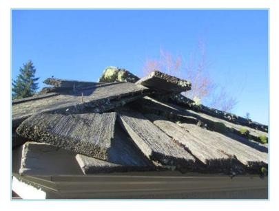
Mailbox kiosk roofs are in fair to poor condition. Damages and missing shingles noted. Some vehicle damage likely.
