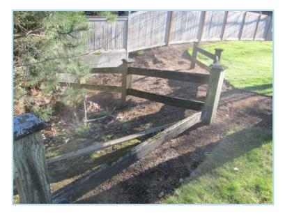
Split rail fencing is in fair to poor condition. Areas of prior repair and damage noted. Although rustic looking by design, this type of fencing will eventually need to be replaced due to constant weathering and exposure. Inspect regularly and repair as needed from operating budget. Plan for regular intervals of replacement at roughly the time frame indicated below.
