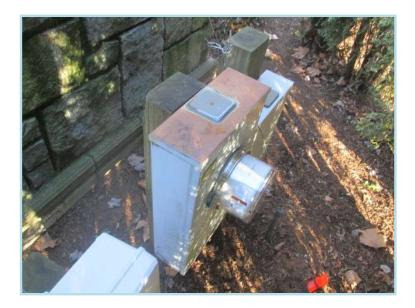
Fair condition noted. Small Circuit breaker panels and meter sockets installed onsite for the common area irrigation and lighting systems. These are located behind some of the monuments. Anticipate the need for eventual replacement of these panels as they are exposed to the elements and the enclosures will eventually corrode. Cost for each location to modernize.
