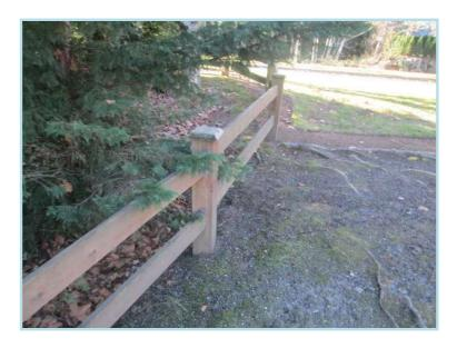
Approx. 50 linear feet of the spit rail fence at NE 30th Ct. has recently been replaced. Although rustic looking by design, this type of fencing will eventually need to be replaced due to constant weathering and exposure. Inspect regularly and repair as needed from operating budget. Plan for regular intervals of replacement at roughly the time frame indicated below.
