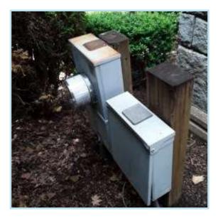
Fair condition noted. Small Circuit breaker panels and meter sockets installed onsite for the common area irrigation and lighting systems. These are located behind some of the monuments. Anticipate the need for eventual replacement of these panels as they are exposed to the elements and the enclosures will eventually corrode. Cost for each location to modernize.
