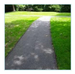
Asphalt pathways at park were reportedly replaced in 2018 for approx. \$33,326. As routine maintenance, keep surface clean, repair cracks and clean oils stains promptly.
