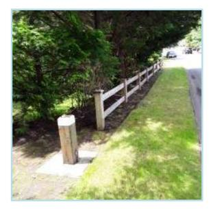
Approx. 50 linear feet of the spit rail fence at NE 30th Ct. has recently been replaced. Although rustic looking by design, this type of fencing will eventually need to be replaced due to constant weathering and exposure. Inspect regularly and repair as needed from operating budget. Plan for regular intervals of replacement at roughly the time frame indicated below.
