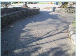
Located at the Circle Park. We recommend budgeting for replacement at the timeframe indicated as these sand set paver systems will typically become uneven with time due to settling, root intrusion, drainage issues and use.
