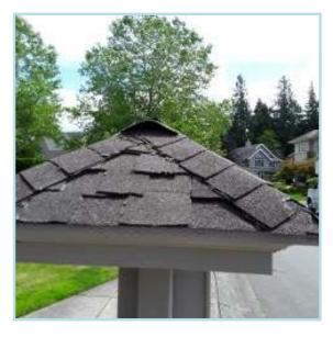
Mailbox kiosk roofs are in fair to poor condition. Damages and missing shingles noted. Some vehicle damage likely.
