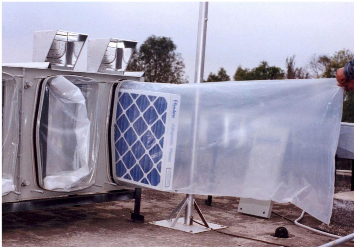
Cobeal's BIBO filter housings for fluid or gasket seal primary filters are side-loading filter housings which have been designed to meet the air filtration needs of industries and research facilities that handle dangerous, toxic, biological or carcinogenic material. To minimize exposure to harmful contamination while replacing used filters, the housing incorporates a ribbed BIBO ring, over which a heavy-duty plastic filter bag is attached (see left).
