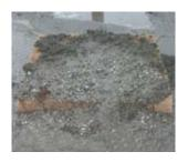
Inlet Filter will collect a lot of sediment. Clean Inlet Filter while mounted on the grate, even if ponded water surrounds the inlet. This unique feature ensures all water entering the grate is filtered. Sweep sides and top of Inlet Filter to remove sediment and debris after each rain event.
