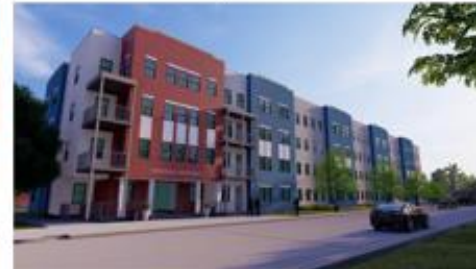
Woodring Apartments Phase I Lake Charles, LA 70 Apartments
