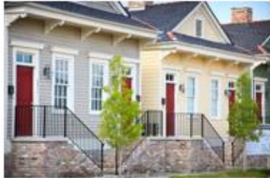
Liberty Place Apartments New Orleans, LA 35 Apartments
