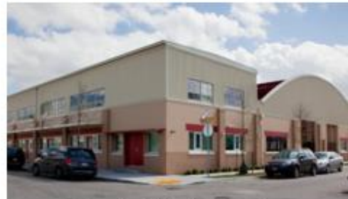
Bywater Art Lofts Phase II New Orleans, LA 30 Apartments
