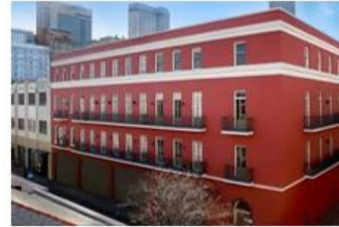
DH Holmes Apartments New Orleans, LA 97 Apartments
