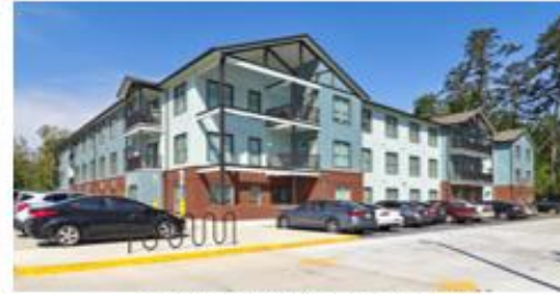
Hammond Station Apartments Hammond, LA 67 Apartments
