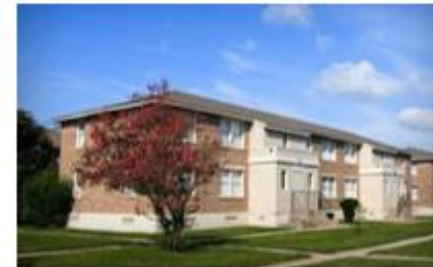
Palmetto Apartments New Orleans, LA 124 Apartments
