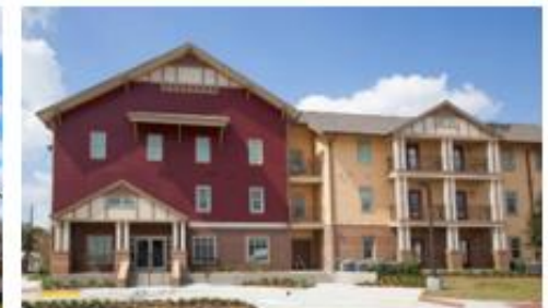
Barataria Station II Houma, LA 43 Apartments
