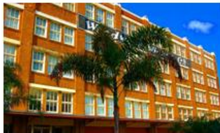
Woodward Lofts New Orleans, LA 192 Apartments
