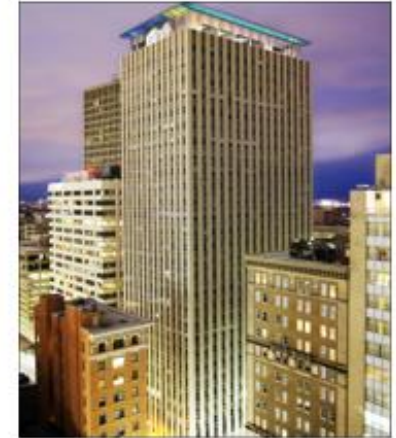
The Strand Apartments New Orleans, LA 192 Apartments
