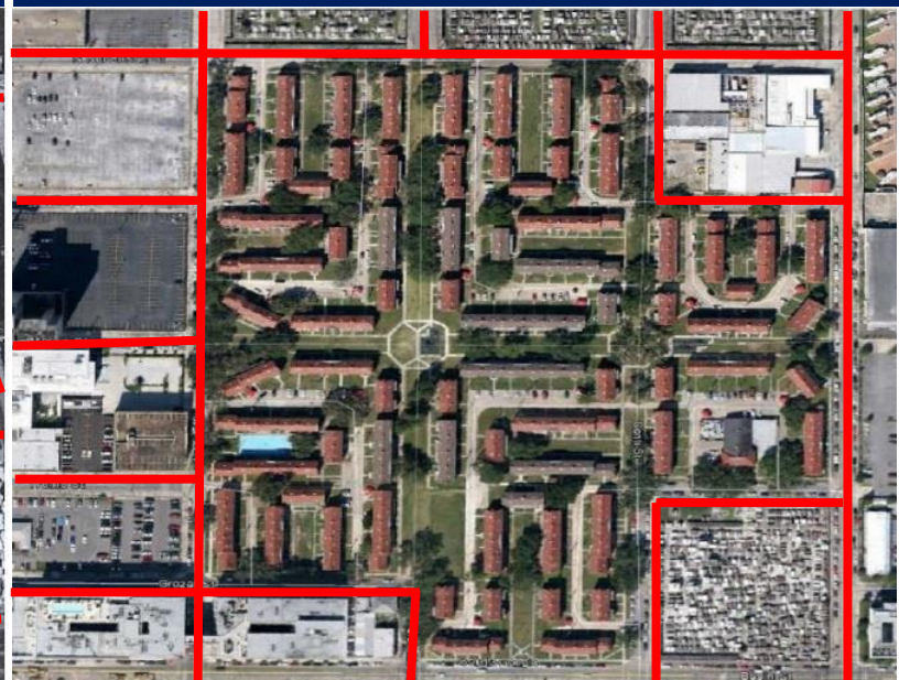
Iberville Housing Project: Interconnecting Street Grid Demolished
