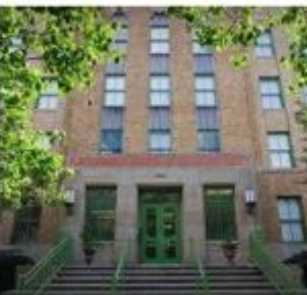
Flint-Goodridge Apartments New Orleans, LA 89 Apartments
