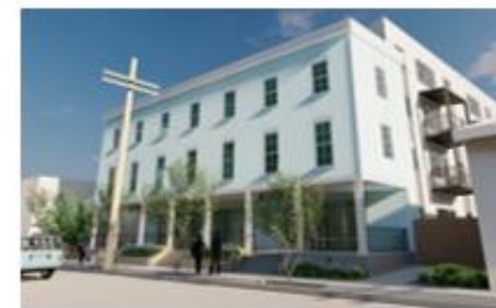
St. Bernard Circle New Orleans, LA 51 Apartments
