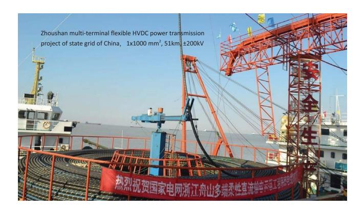
ZTT HVDC submarine cable is based on XLPE insulation, used on VSC (Voltage-Source Converter) system. Up to now, we can produce up to  $\pm 320 kV$  HVDC.
