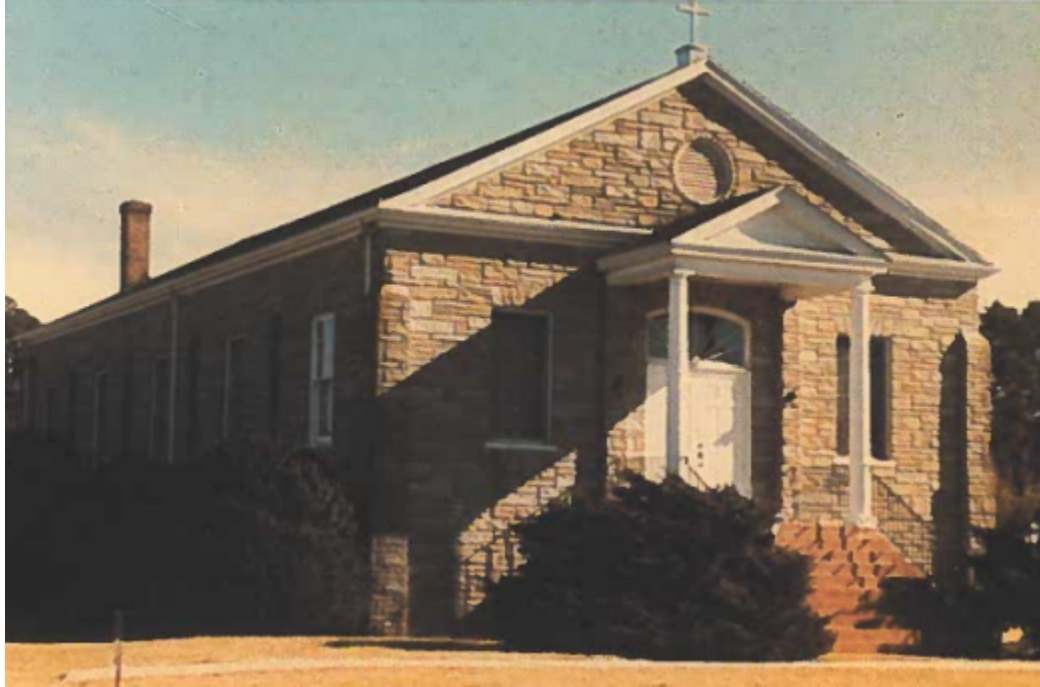
The church just before the addition.
