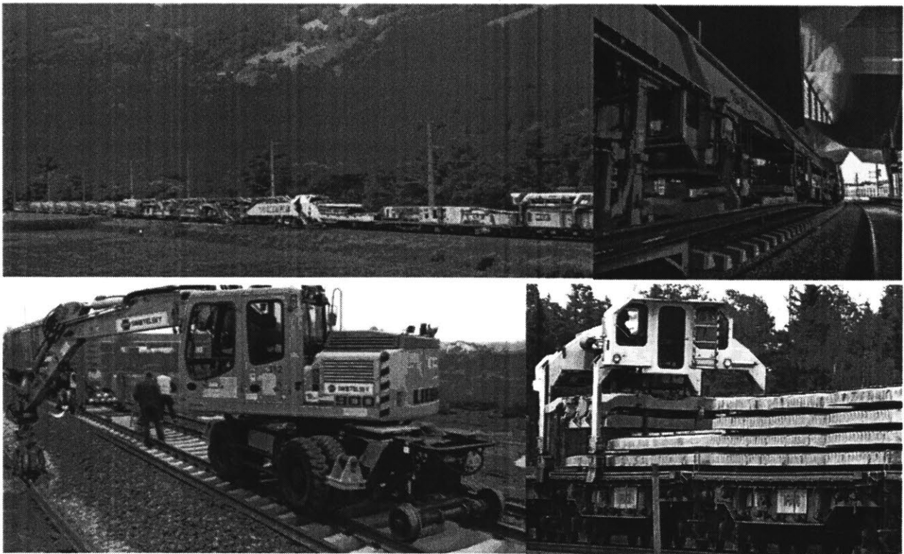
Figure 19: (Top, Left) A rolling stock machine used to make or replace railroads. The various sections of the train accomplishes operations like ground preparation, ballast pouring, foundation installation, rail pulling, ballast tamping, and rail welding. The existence of these machines allows convenient maintenance and repair of railways. (Top, Right) A view of the same rolling stock railroad-building machine installing concrete foundations at a train station. (Bottom, Left) A commonly found bogie-mounted backhoe capable of fluid operation on and around railroads. (Bottom, Right) A gantry crane capable of traveling from car to car to shuttle pre-cast concrete railroad foundations along the length of a railroad building machine, from “sleeper cars,” to where the pieces are being installed.
