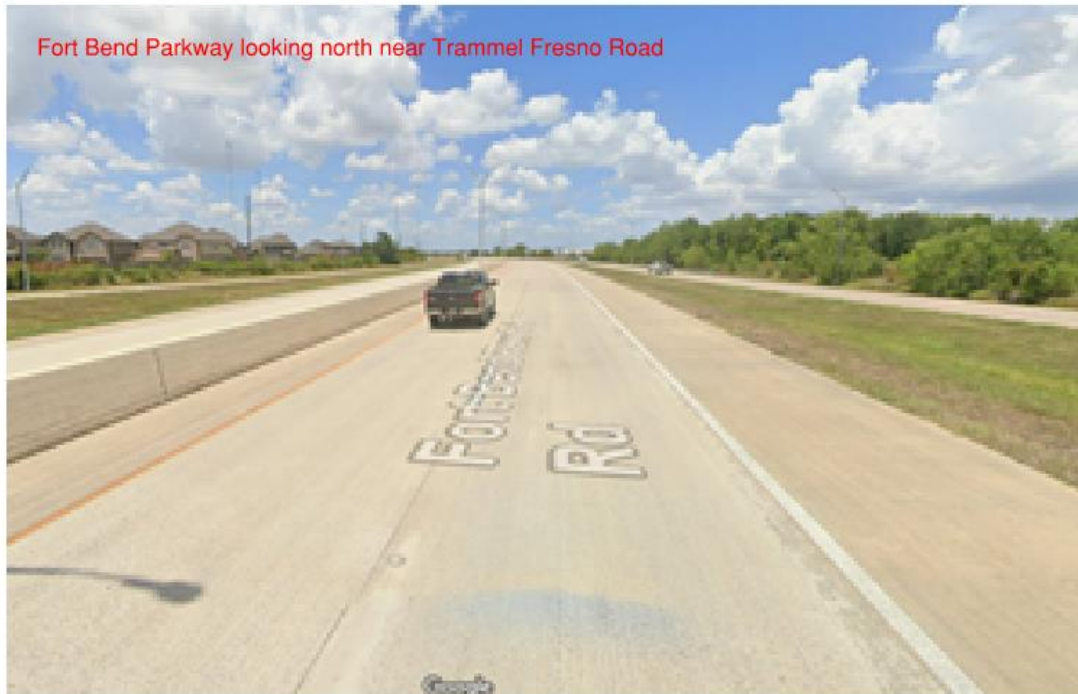
Fort Bend Parkway looking north near Trammel Fresno Road
