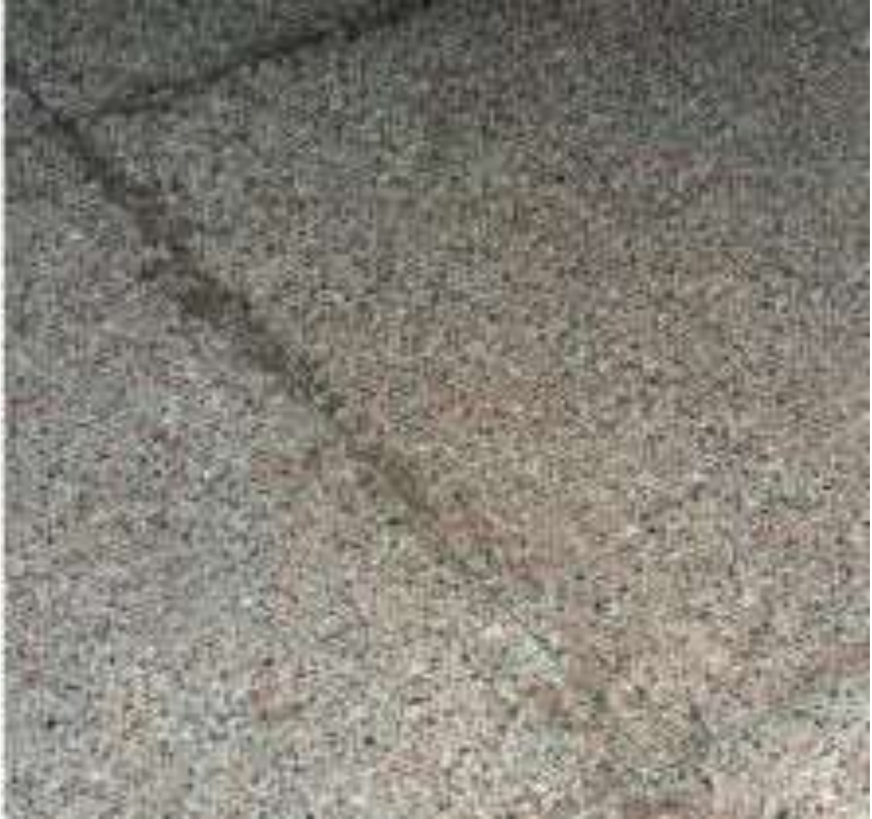
Photo 2 - Moisture Vapor Transmission through Polyacrylate Terrazzo Joints
