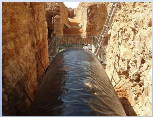
• SWCC Jubail Pump Station - EPWTS Dn1500 Emergency Connection Line. (old materials made it usable by sandblasting, painting and fittings fabrication)
