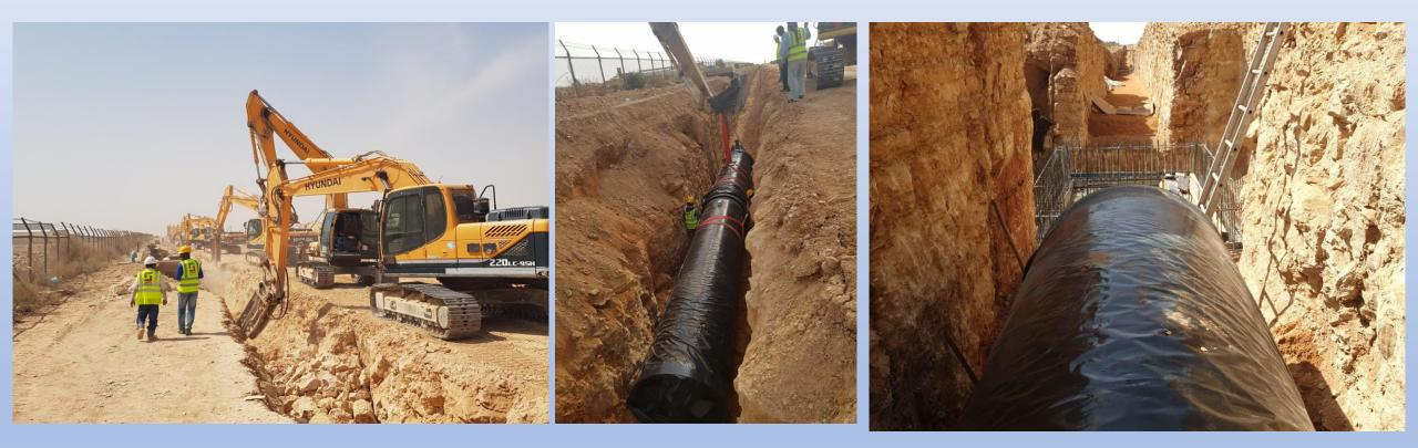
• SWCC Jubail Pump Station - EPWTS Dn1500 Emergency Connection Line. (old materials made it usable by sandblasting, painting and fittings fabrication)
