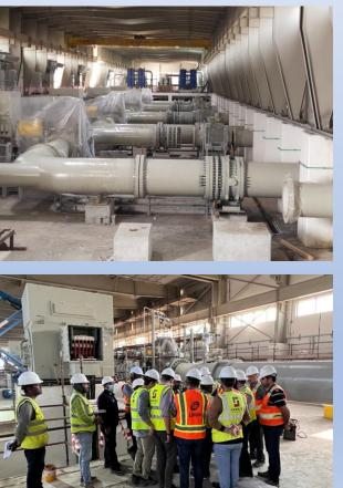
• Neom WTS. The scope includes all the station piping, pump station, surge vessels and air compressor installation at Duba PS1 and Sharma HPR.
