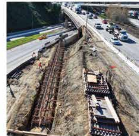
Northbound SR-57 connector bridge widening over Golden Springs Drive
