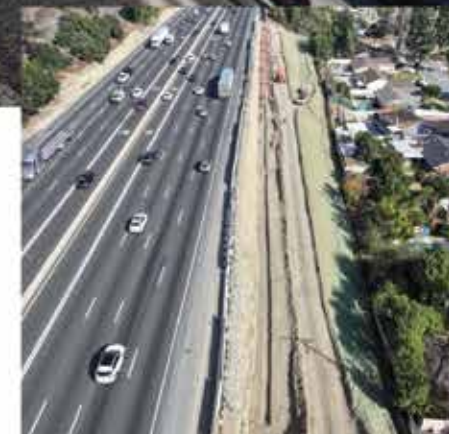
Retaining wall construction along eastbound SR-60
