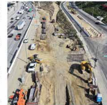
Relocation of sanitary sewer line
