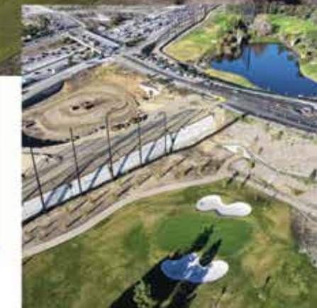
Embankment for Grand Ave on- and off-ramp
