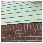
There were unsealed joints in the hardboard siding. We recommend the joints be caulked or sealed. This is a part of routine homeowner maintenance.
