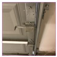
The overhead garage door lock has not been disabled. This is considered an entrapment hazard based on the state regulated standards of practice
