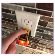
Though the kitchen was equipped with GFCI style receptacles, when tested some of the receptacles did not trip, and therefore, lack GFCI protection
