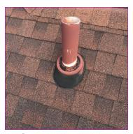
There were exposed fasteners at Some flashings were incorrectly installed & do not fully serve their intended purpose.
