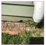
Sections of the hardboard siding were damaged
