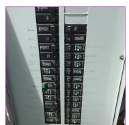
Breaker panel was not labeled or was partially labeled. This is a deficiency
