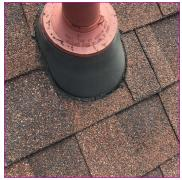
One or more flashing were not properly sealed at the time of inspection
