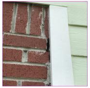
Gaps in the hardboard siding were observed at one or more of the pipe and/or vent penetrations. We recommend all such gaps be sealed or plugged in the course of routine property maintenance
