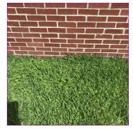
Soil height close to the exterior facade on part of the structure. This is a path for insects & moisture to travel to enter the home.
