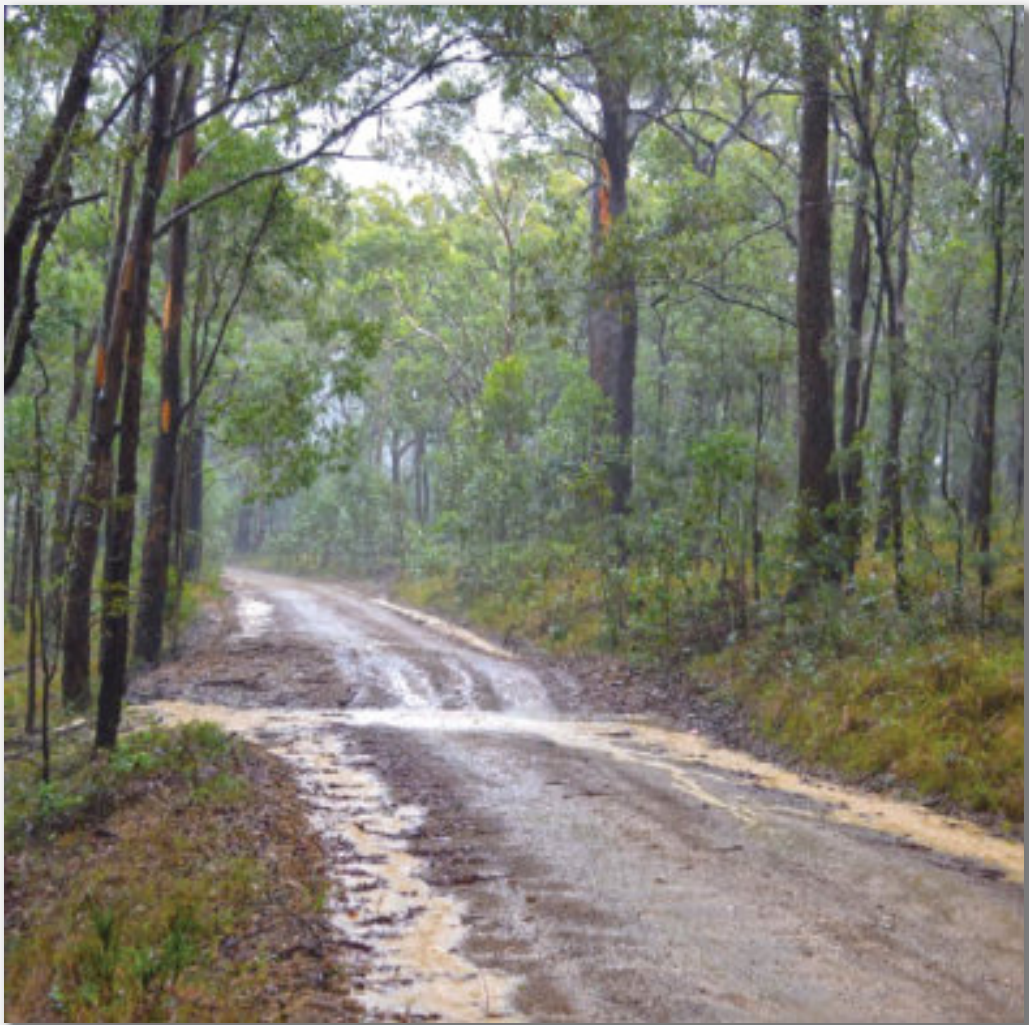
Above. Fire trails require passing bays and turning bays dependent on the category of vehicle/trail. Below. A well formed fire trail with longitudinal table drains and a cross bank allowing upslope water to drain across the trail with the minimum of erosion. (Images from NSW RFS Fire Trail Design, Construction and Maintenance Manual)
