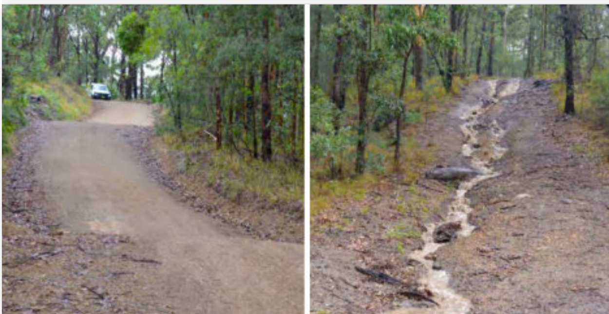
Two examples of fire trails: one well maintained and one suffering from erosion. (Image by Soil Conservation Service's NSW RFS Fire Trail Manual)
