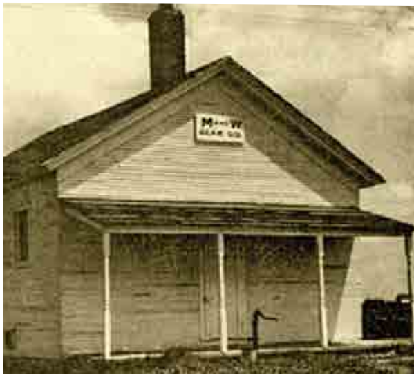
Rockford Rural schoolhouse which was the first factory of M&W Gear
