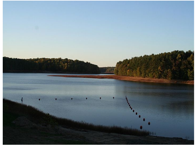
Drinking water reservoir
