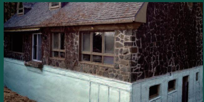
⬡ Heatlok Soya is ideal for insulating old concrete or stone foundations from the exterior.
