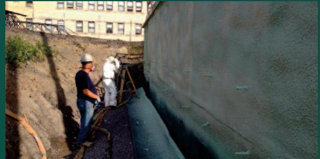
⬡ The photo on the left shows a bituminous coating applied directly over spray polyurethane foam. The photo on the right shows a drainage membrane that will be lifted in front of the spray polyurethane foam as the soil is backfilled.
