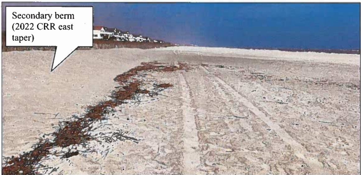
Figure 2-23 (B). April 2022 photograph near Station 40+00 looking east. Note newly constructed secondary berm along east taper of CRR which ties in with the 2022 LWFIX project at this location.
