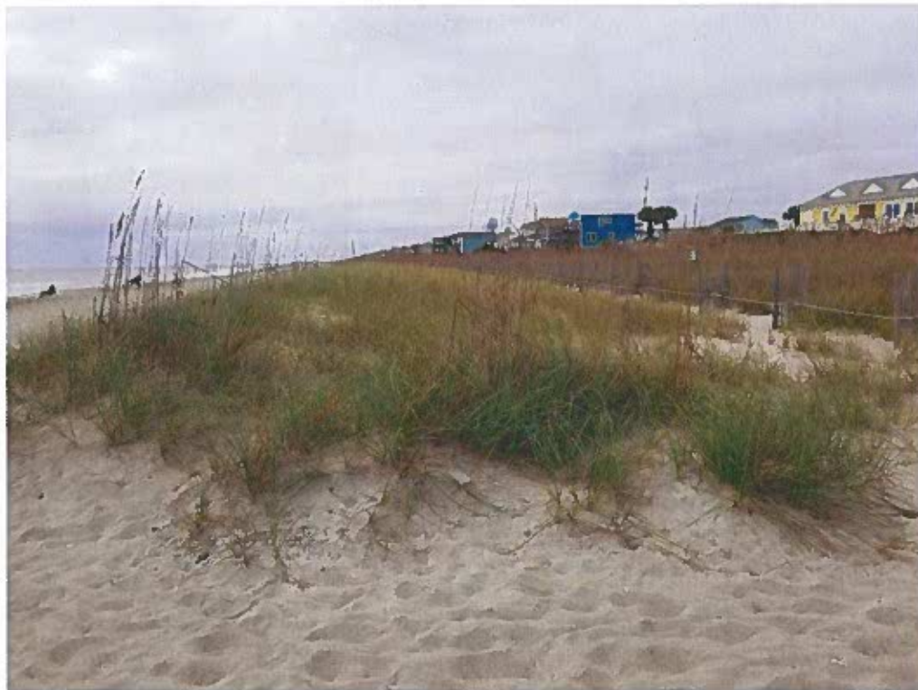
Figure 2-31 October 2024 between Station 60+00 and Station 70+00 showing plant growth ~2.5-year post CRR along newly constructed secondary berm (and after Hurricane Ian in 2022).
