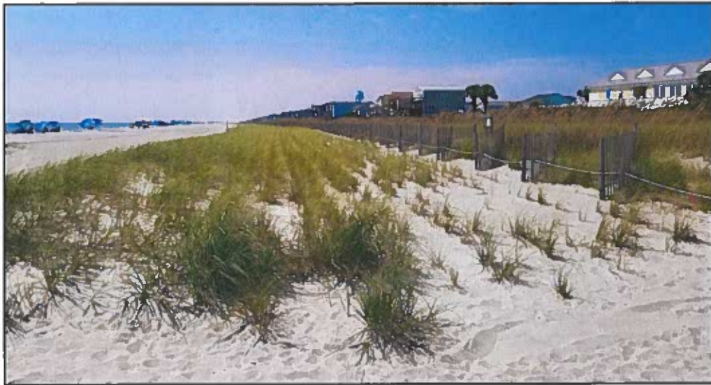
Figure 2-30. September 2023 between Station 60+00 and Station 70+00 showing plant growth ~1.5-year post CRR along newly constructed secondary berm (and after Hurricane Ian).
