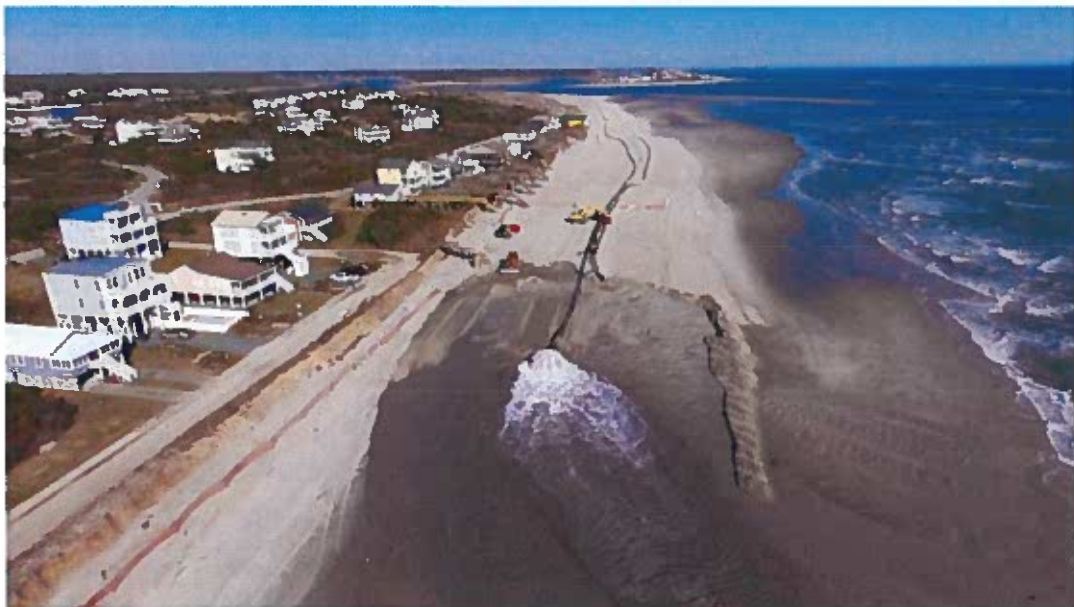
Figure 2-16. Holden Beach POA Aerial Photograph taken during 2017 Eastern Reach Project Construction (pumping just west of Station 30+00).
