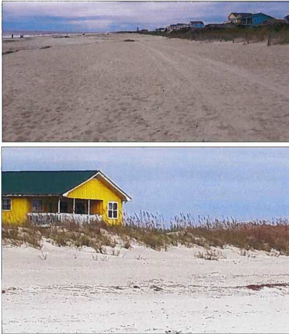
Figure 3-6. Recent Photographs of East End Beach Conditions Taken between Stations 20+00 and 30+00 Looking West (Upper Photo) and East (Lower Photo). ~2.5-year post 2022 LWIFX Placement Showing Wide Beach Present in What Is Typically an Erosional Hotspot Area (Photos Taken October 2024).
