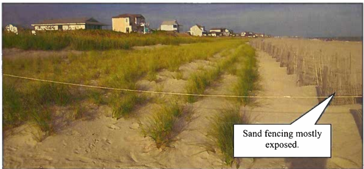
Figure 2-28 (A). Sand Fencing along the Seaward Edge of the Starter Dune for the Central Reach Project at Station ~60+00 Showing Planted Dune Vegetation. (ATM photo, taken August 2018).
