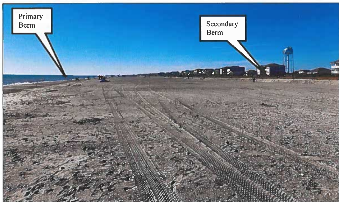
Figure 2-9 (A). CRR Post-Construction Near Station 80+00 (ATM photo taken 02/10/2022).
