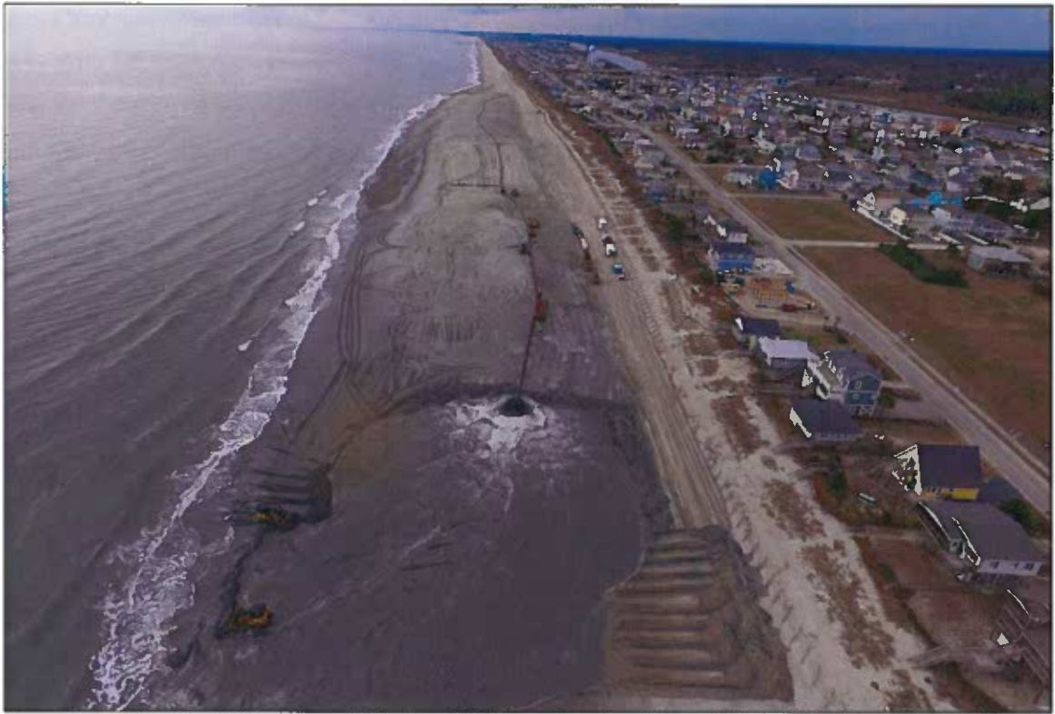
Figure 2-7 (A). Aerial Photograph During CRR Construction, Photo Taken Near East Taper, ~Station 40+00, Looking West (ATM Drone Photo 01/20/22).
