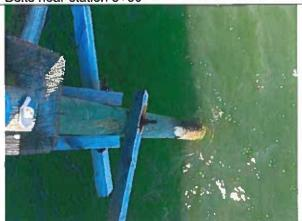
Photo 35: Typical Pile Flaking and Gouging near station 5+75
