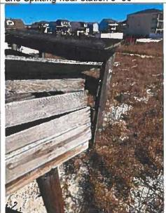
Photo 5: Typical Railing Detachment and Failure near station 0+90
