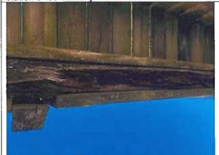
Photo 65: Typical Rotting Joist near station 0+90 Balcony
