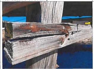
Photo 69: Cross Bracing Checking and Splitting near station 1+00
