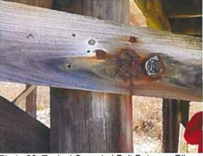
Photo 62: Typical Corroded Bolt Between Pile and Bracing Member near station 0+75
