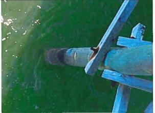
Photo 48: Typical Checking in Bracing near station 7+00
