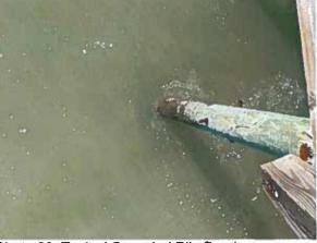
Photo 20: Typical Corroded Pile Bracing Connection with Missing Brace near station 3+75
