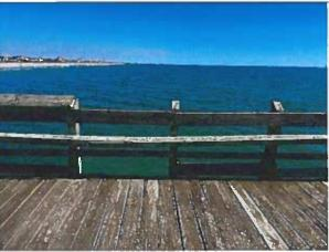
Photo 50: Typical Missing Top Rail and Toe Boards near station 7+25
