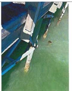
Photo 30: Typical Corroded Bracing and Pile Connection near station 4+25
