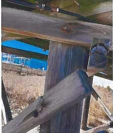
Photo 68: Typical Bracing Member Checking and Splitting near station 0+90 Balcony
