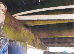
Photo 60: Typical Joist Notching at Support near station 0+75
