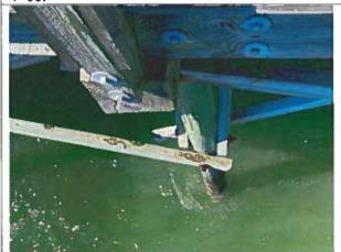
Photo 27: Typical Corroded Bracing Connection near station 4+25
