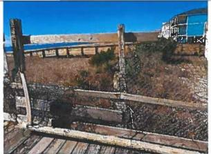
Photo 1: Typical Railing and Fence Damage near station 0+10
