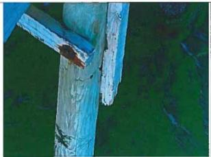
Photo 55: Typical Pile Gouging and Flaking near station 7+50
