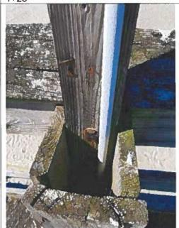
Photo 9: Typical Utility Conduit Timber Casing near station 2+00
