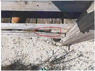
Photo 8: Typical Joist Deterioration near station 1+25
