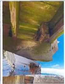
Photo 67: Typical Support Checking and Splitting near station 0+90 Balcony
