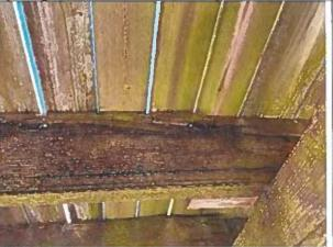
Photo 70: Typical Disconnected and Split Joist near station 1+00
