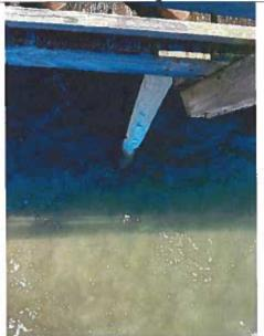
Photo 22: Rail Post Corroded Connection Bolt near station 3+75
