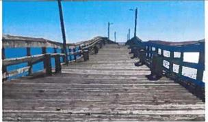
Photo 17: Typical Deck Warping between station 3+25 and station 4+10
