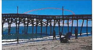
Photo 18: Typical Deck Warping between station 3+25 and station 4+10
