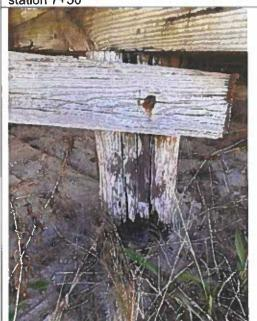
Photo 57: Typical Pile Exterior Rot Deterioration near station 0+00
