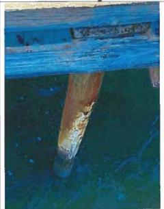
Photo 21: Typical Timber Pile Flaking and Gouging near station 3+75
