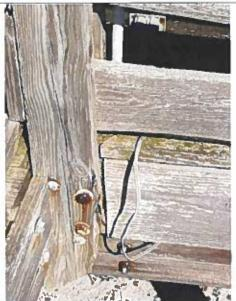
Photo 6: Typical Rail Post Gouging and Connection Bolt Corrosion near station 0+90
