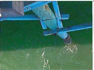
Photo 46: Cracked Pile near station 7+00
