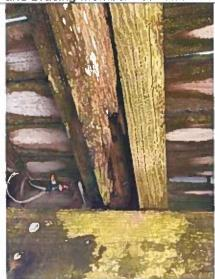
Photo 63: Typical Rotting Joist / Supports near station 0+90 Balcony
