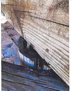
Photo 58: Typical Hollow Pile Deterioration near station 0+00
