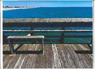
Photo 45: Typical Bench and Missing Toe Boards near station 7+00
