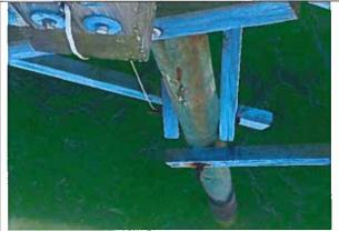
Photo 37: Pile Flaking and Gouging and Bracing Checking near station 6+00
