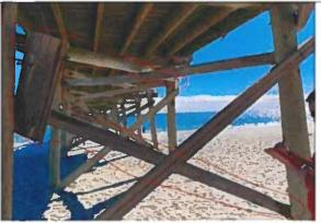
Photo 73: Disconnected Cross Bracing near station 2+25
