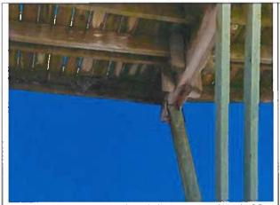
Photo 85: Typical Rotting Joist near station 4+00
