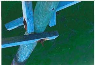
Photo 47: Cracked Pile near station 7+00
