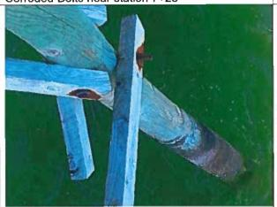
Photo 51: Typical Pile Gouging and Checking near station 7+25
