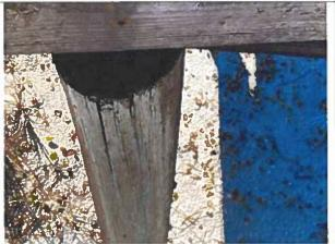
Photo 4: Typical Hollow Pile near station 0+90
