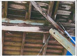
Photo 87: Pile Cap Splicing / Repair near station 4+00
