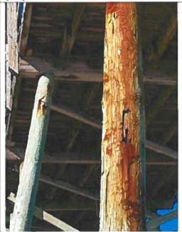
Photo 83: Pile Gouging and Flaking near station 3+75
