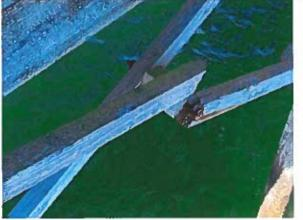
Photo 36: Typical Broken (Disconnected) Bracing near station 6+00
