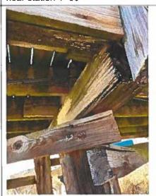
Photo 72: Typical Pile Cap End Rot near station 1+50
