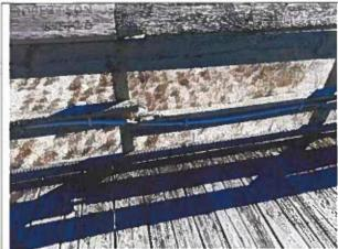
Photo 7: Typical Midrail Separation near station 1+25
