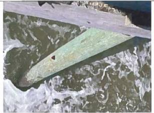
Photo 19: Typical Corroded Pile Bracing
