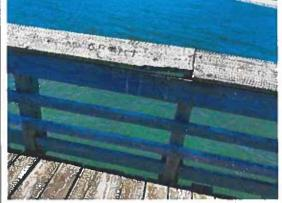
Photo 42: Typical Top Rail Disconnection near station 6+75
