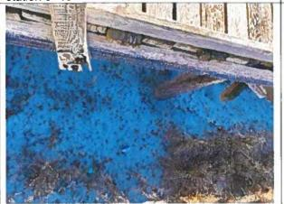
Photo 3: Typical Rail Post Connection Corrosion and Splitting near station 0+90
