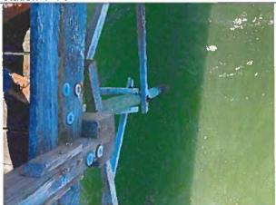
Photo 33: Typical Corroded Bracing Connection Bolts near station 5+00
