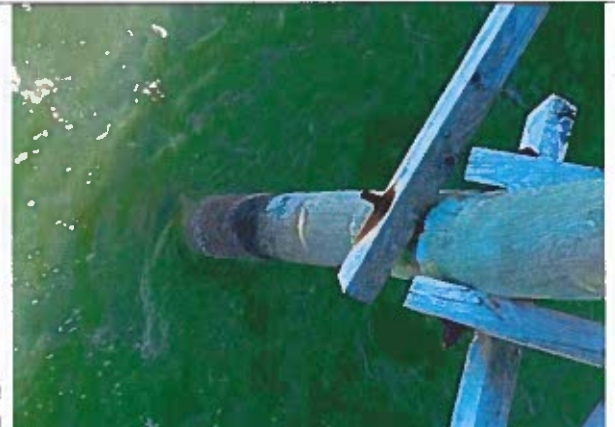
Photo 48: Typical Checking in Bracing near station 7+00
