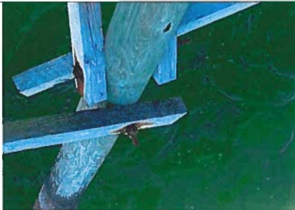
Photo 47: Cracked Pile near station 7+00
