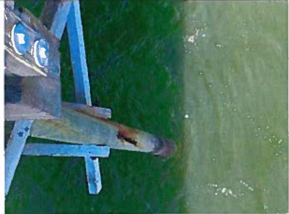
Photo 38: Typical Missing Bracing Member and Corroded Bolt near station 6+25
