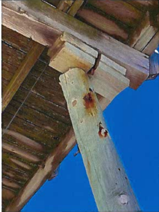
Photo 81: Misaligned Pile Missing Pile / Pile Cap Connection and Missing Bracing near station 3+75
