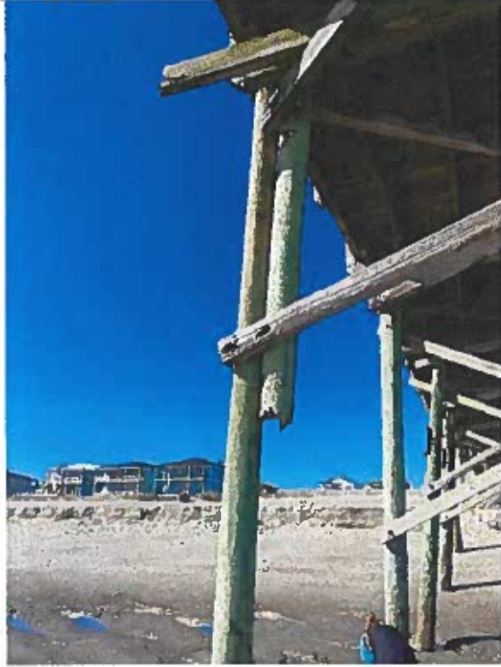
Photo 78: Typical Pile Sistering Repair near station 2+75
