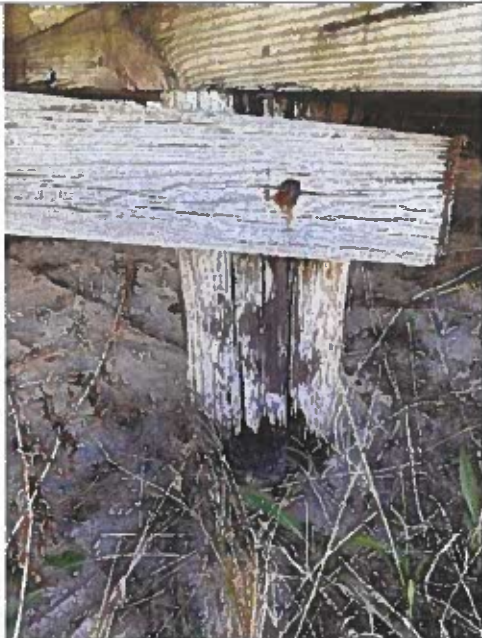
Photo 57: Typical Pile Exterior Rot Deterioration near station 0+00
