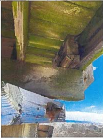
Photo 67: Typical Support Checking and Splitting near station 0+90 Balcony
