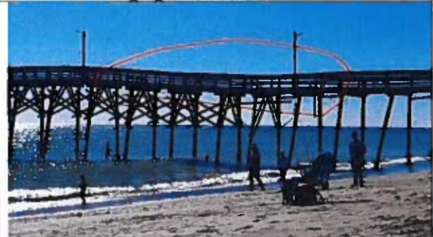
Photo 18: Typical Deck Warping between station 3+25 and station 4+10
