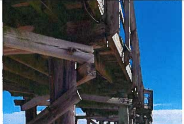
Photo 74: Split / Checked Cross Bracing and Pile Cap End Rot near station 2+25
