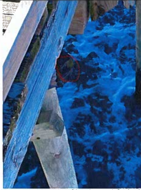
Photo 14: Typical Checks and Splits in the Cross Bracing near station 3+00
