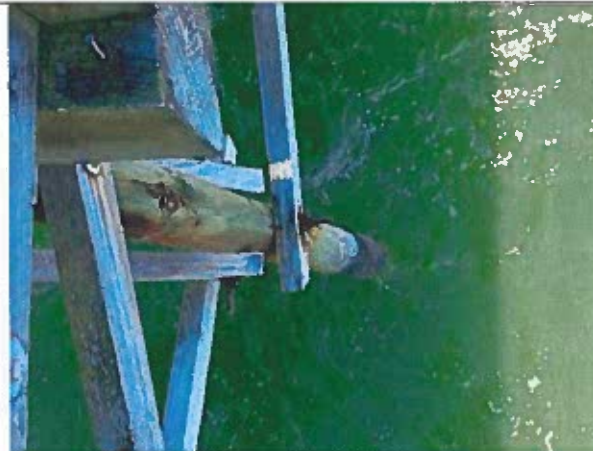
Photo 34: Typical Corroded Bracing Connection Bolts with Pile Gouging near station 5+50
