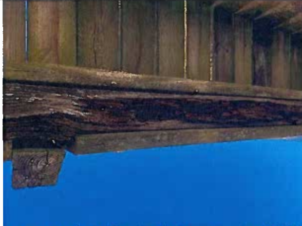
Photo 65: Typical Rotting Joist near station 0+90 Balcony
