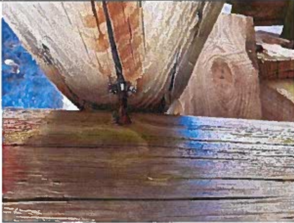
Photo 61: Typical Corroded Bolt Between Pile and Bracing Member near station 0+75
