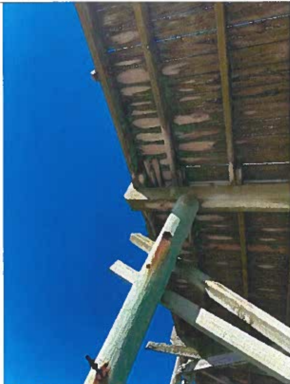
Photo 79: Typical Pile with Missing Cross Bracing and Missing Pile / Pile Cap Connection near station 3+00
