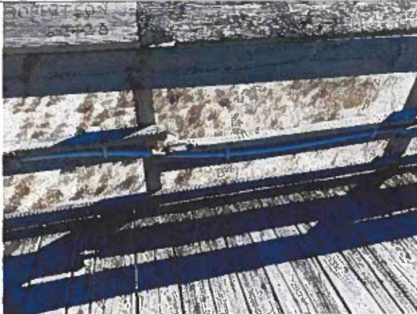
Photo 7: Typical Midrail Separation near station 1+25
