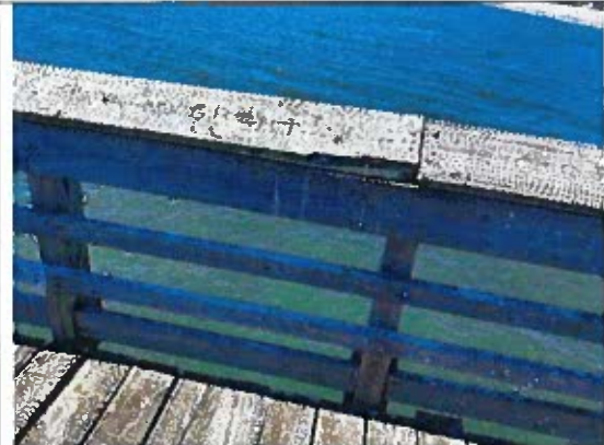
Photo 42: Typical Top Rail Disconnection near station 6+75
