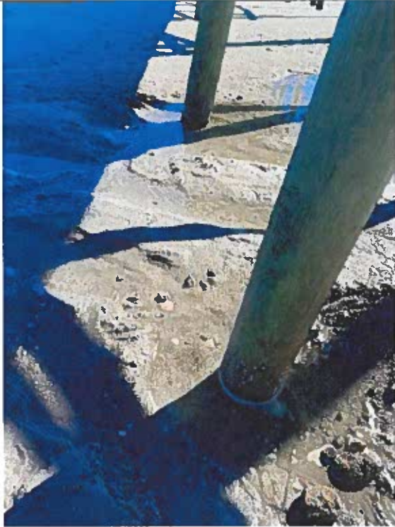
Photo 77: Typical Pile Marine Growth and Localized Scour in the Tidal Zone near station 2+75
