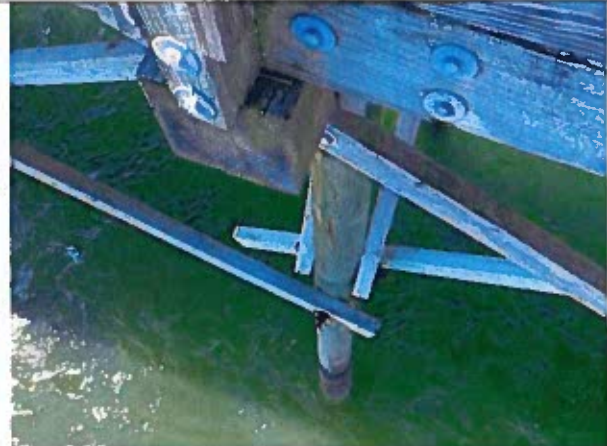
Photo 40: Pile Checking and Gouging near station 6+50
