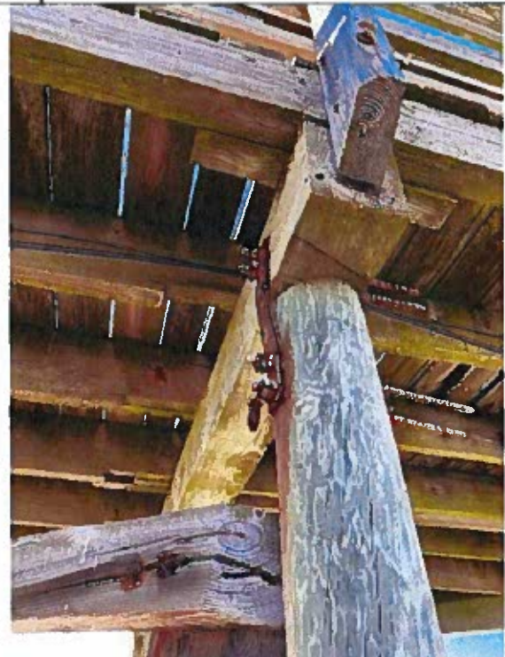
Photo 76: Corroded Pile / Pile Cap Connection and Cross Bracing Connection near station 2+50
