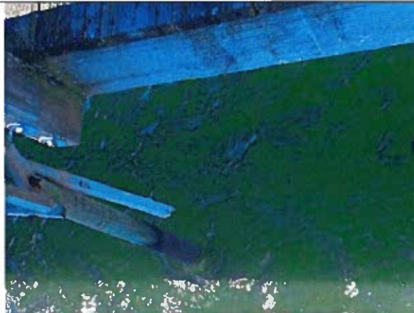
Photo 39: Typical Broken Bracing Member near station 6+50
