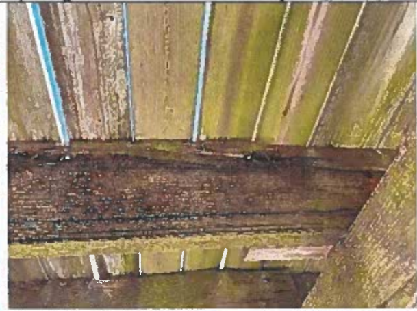
Photo 70: Typical Disconnected and Split Joist near station 1+00
