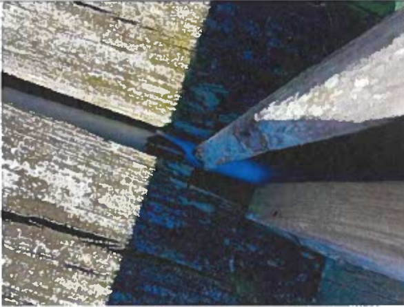
Photo 31: Typical Conduit Housing Damage near station 4+75
