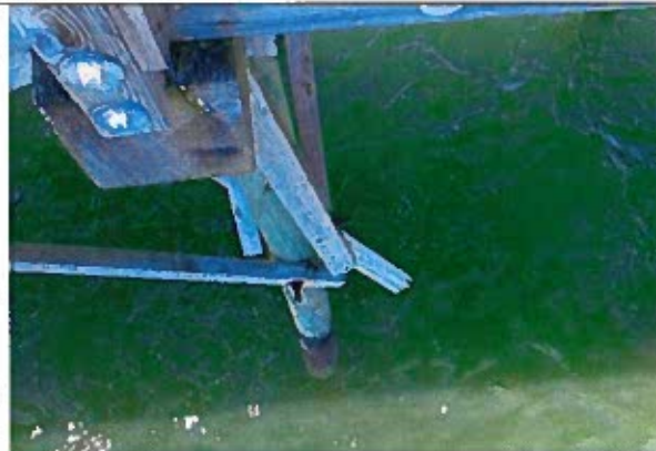
Photo 41: Typical Broken Bracing Member and Pile Cap Checking near station 6+75
