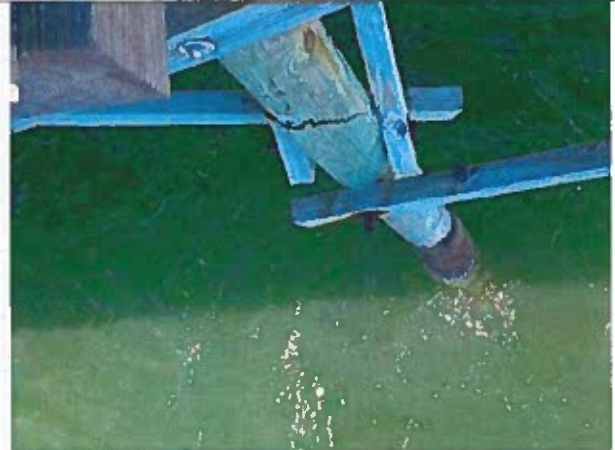
Photo 46: Cracked Pile near station 7+00
