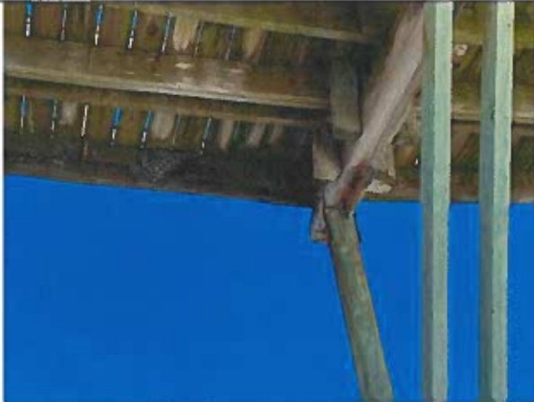
Photo 85: Typical Rotting Joist near station 4+00
