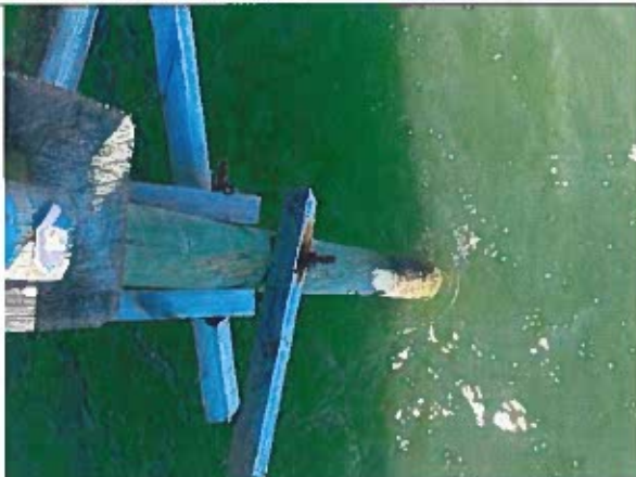
Photo 35: Typical Pile Flaking and Gouging near station 5+75
