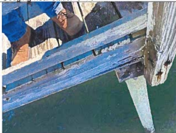
Photo 23: Corroded Connection and Checking at Rail Post and Timber Pile Cap Beam. Pile with Missing Brace and near station 4+00
