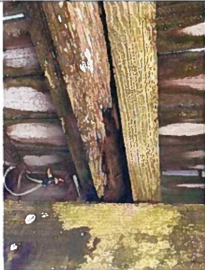
Photo 63: Typical Rotting Joist / Supports near station 0+90 Balcony
