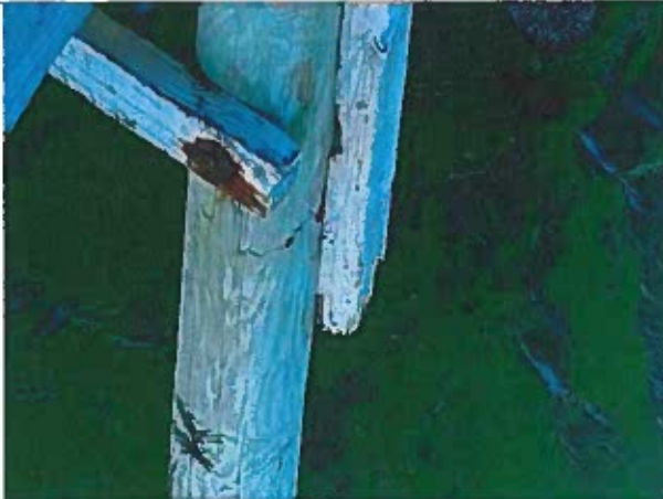
Photo 55: Typical Pile Gouging and Flaking near station 7+50
