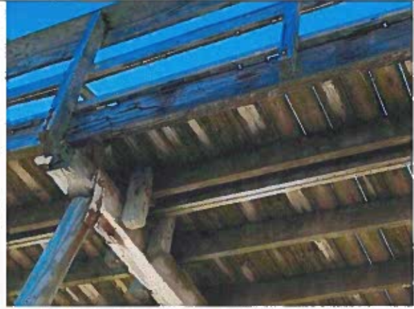
Photo 86: Rotting Joist and Pile Cap End Rot near station 4+00
