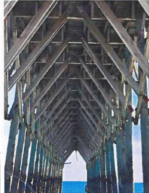
Photo 90: Broken Bracing and Corroded Connection Bolts Beyond station 4+00
