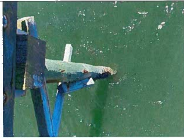
Photo 52: Typical Broken and Missing Bracing Member and Corroded Bolts near station 7+50
