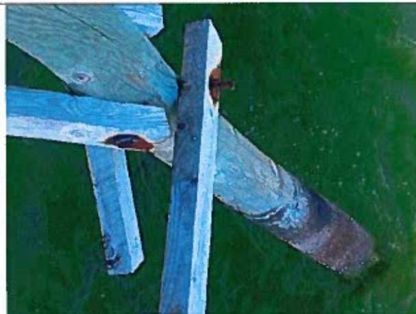
Photo 51: Typical Pile Gouging and Checking near station 7+25
