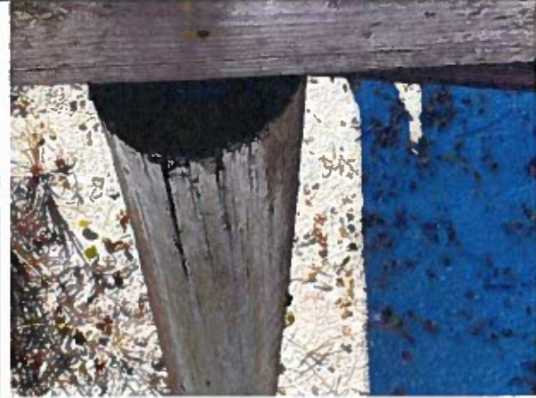
Photo 4: Typical Hollow Pile near station 0+90
