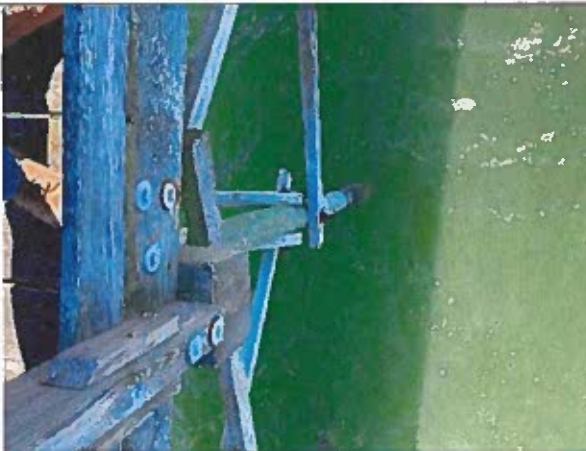
Photo 33: Typical Corroded Bracing Connection Bolts near station 5+00
