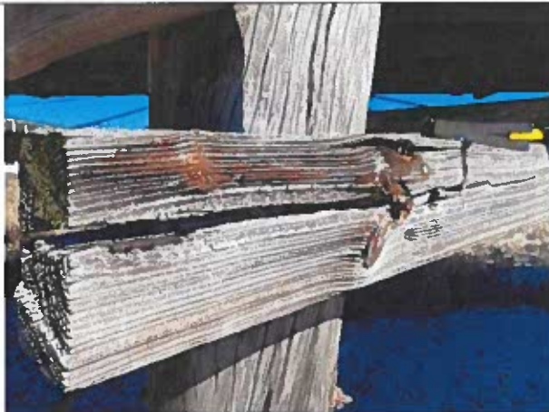
Photo 69: Cross Bracing Checking and Splitting near station 1+00
