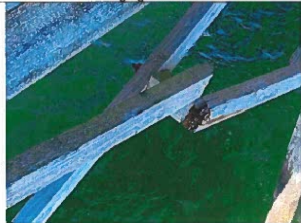
Photo 36: Typical Broken (Disconnected) Bracing near station 6+00
