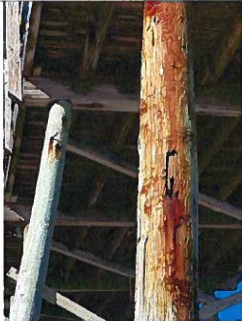
Photo 83: Pile Gouging and Flaking near station 3+75
