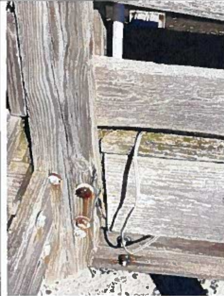
Photo 6: Typical Rail Post Gouging and Connection Bolt Corrosion near station 0+90
