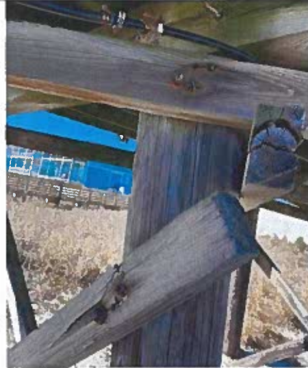
Photo 68: Typical Bracing Member Checking and Splitting near station 0+90 Balcony
