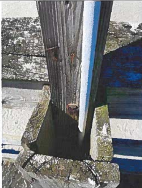
Photo 9: Typical Utility Conduit Timber Casing near station 2+00
