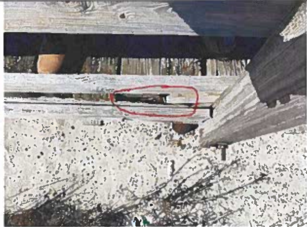
Photo 8: Typical Joist Deterioration near station 1+25
