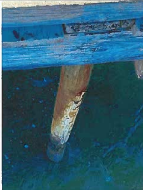
Photo 21: Typical Timber Pile Flaking and Gouging near station 3+75
