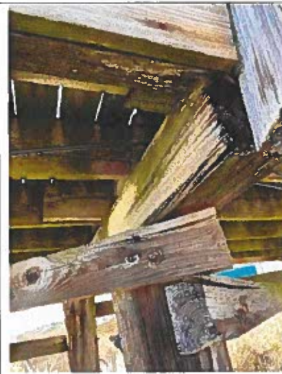
Photo 72: Typical Pile Cap End Rot near station 1+50
