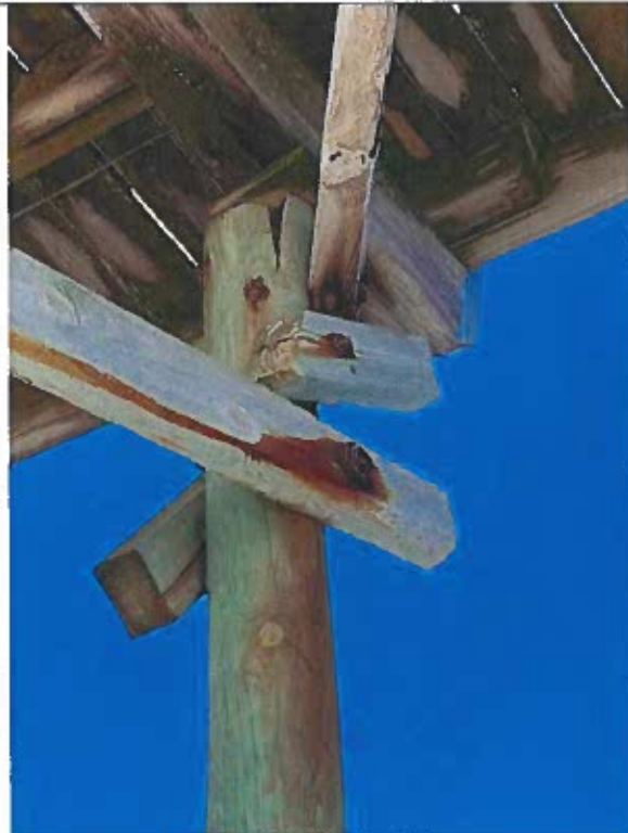
Photo 80: Split Pile Head with missing Pile / Pile Cap Connection Tie near station 3+50
