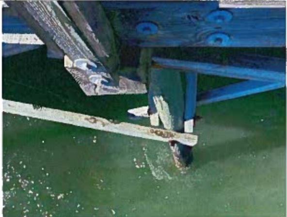
Photo 27: Typical Corroded Bracing Connection near station 4+25
