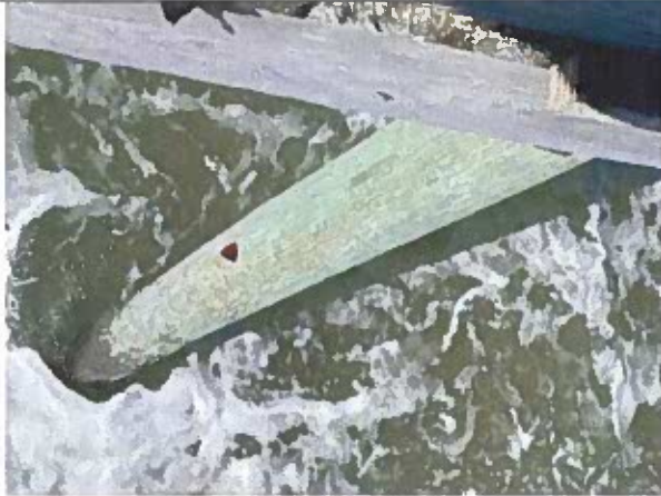
Photo 19: Typical Corroded Pile Bracing Connection with Missing Brace near station 3+25
