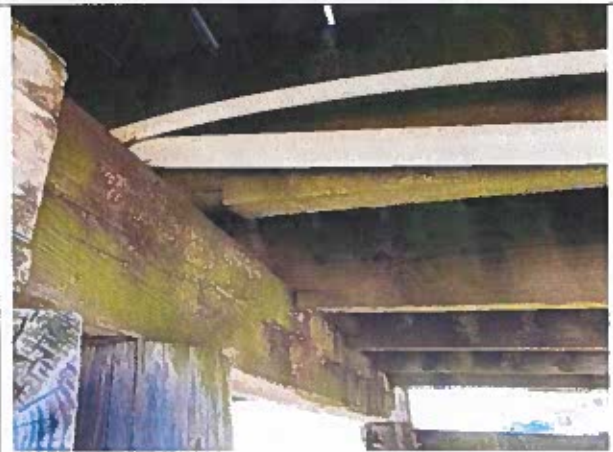
Photo 60: Typical Joist Notching at Support near station 0+75
