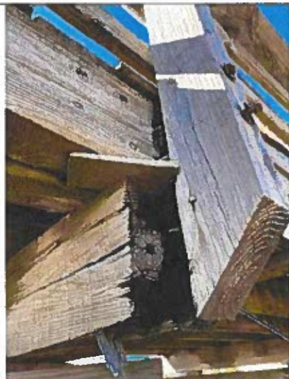
Photo 71: Typical Pile Cap End Rot and Detached Railing Post near station 1+25
