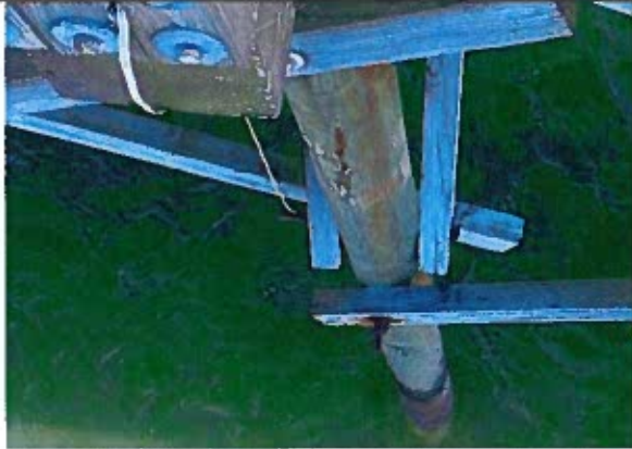
Photo 37: Pile Flaking and Gouging and Bracing Checking near station 6+00
