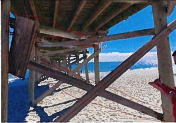
Photo 73: Disconnected Cross Bracing near station 2+25
