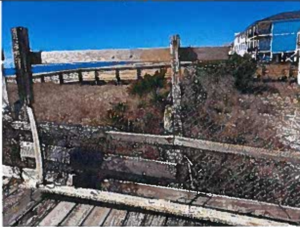
Photo 1: Typical Railing and Fence Damage near station 0+10
