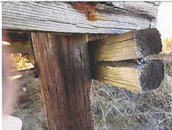
Photo 59: Typical Cross Bracing Checking and Splitting near station 0+50
