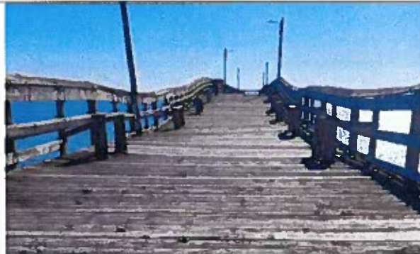
Photo 17: Typical Deck Warping between station 3+25 and station 4+10
