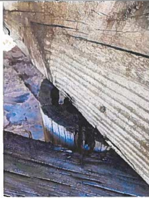
Photo 58: Typical Hollow Pile Deterioration near station 0+00
