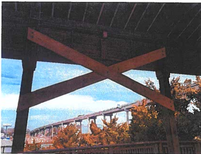
Photo 7 – Temporary X Bracing recently installed
