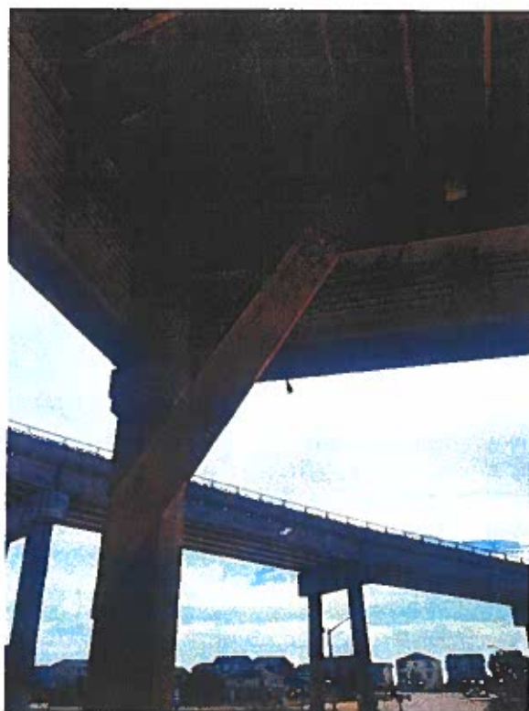
Photo 8 – Temporary Column Bracing recently installed
