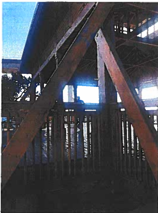
Photo 2 – Rear left side temporary bracing
