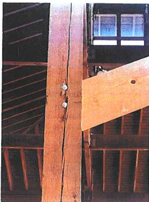
Photo 9 – Temporary Column Bracing recently installed with split column
