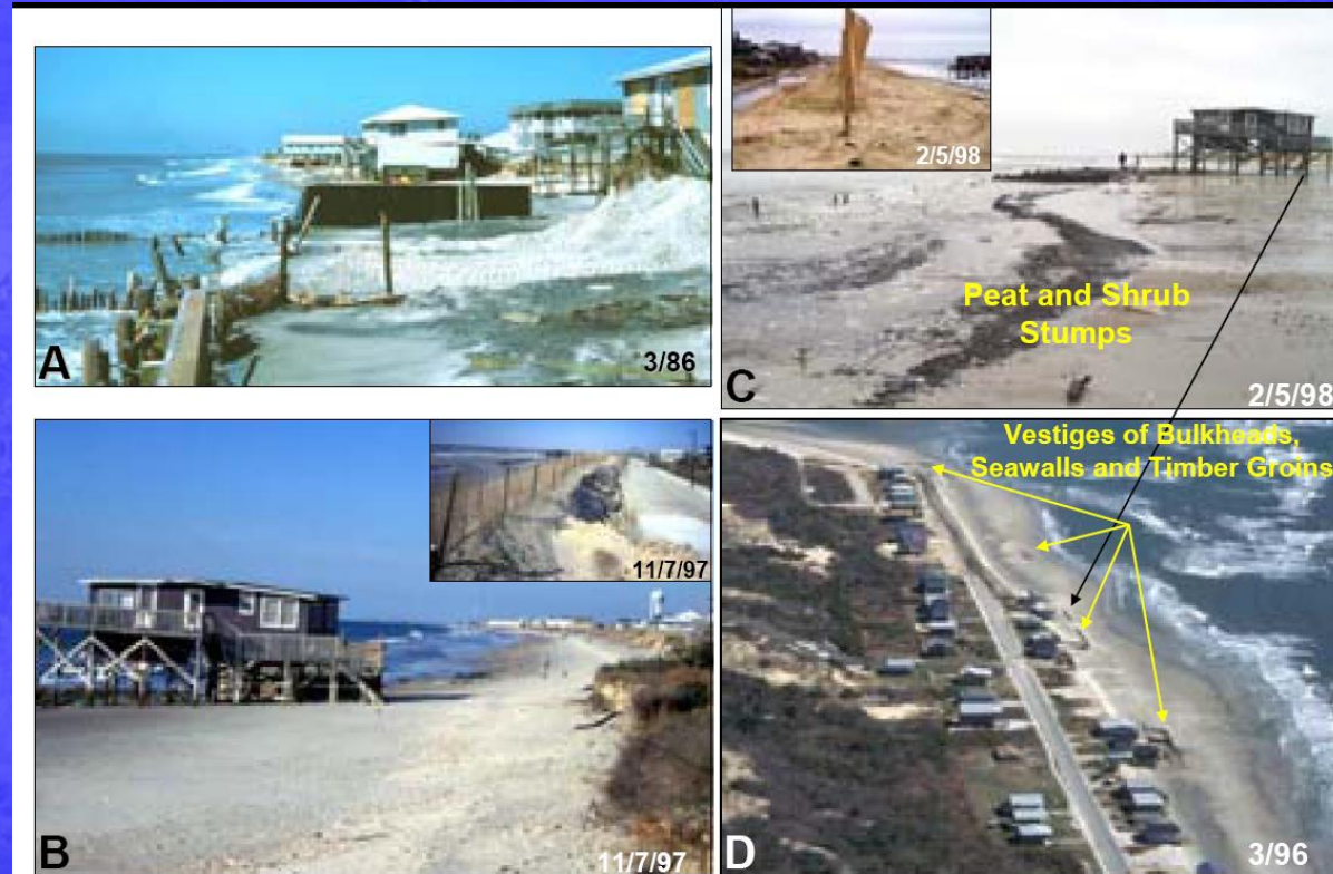
Figure 39. Photographs of the eastern portion of Holden Beach. A. West view (3/86) of eroding shoreline and houses stranded on recreational beach. Note bulkheads, timber groins and vestiges of seawalls that litter the beach. The eastern portion of Holden Beach shoreline near the inlet has been a chronic erosion zone since the late 1970s. B. West view (11/7/97) of same area in "A" retreat of the shoreline, removal of all but one home and a refurbished dune/dike composed of truck hauled sand. C. Aerial photograph of house on beach and peat exposure. Insert depict dike along road. D. Aerial photograph depicting shoreline and chronic erosion zone. Note the homes fronted by bulkheads and remnants of those destroyed.
