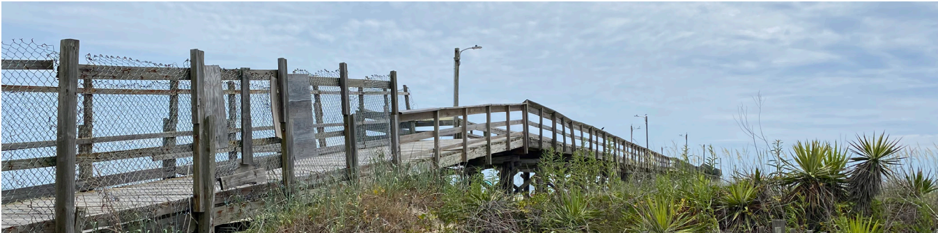
Pier – current conditions
