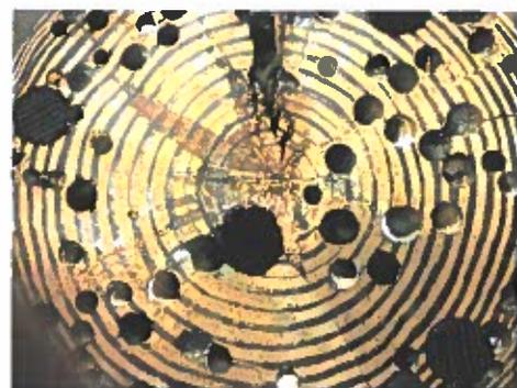
With growth cleaned / scraped on the pile, the small holes noted on the left would note a potential for teredo and lead to taking some cores into the pile to detect deterioration (holes could be plugged after inspection).
