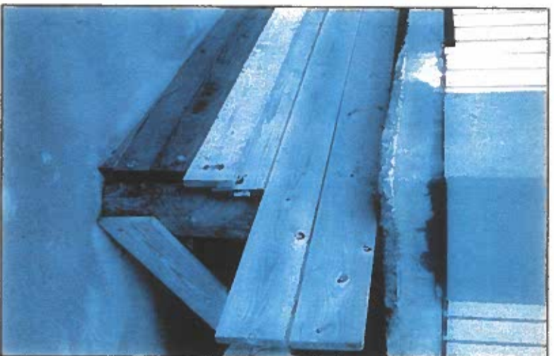
Figure 25: Shore-parallel timbers attached to a pile foundation that were intended to act as a bulkhead but constituted an obstruction and are not permitted
