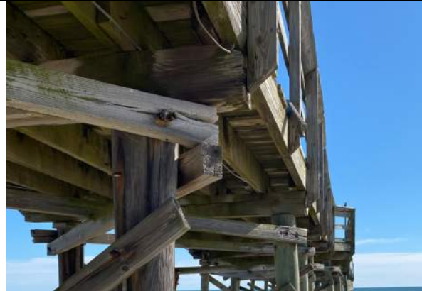
Photo 74: Split / Checked Cross Bracing and Pile Cap End Rot near station 2+25
