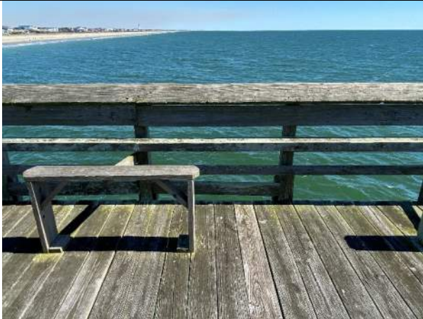
Photo 45: Typical Bench and Missing Toe Boards near station 7+00
