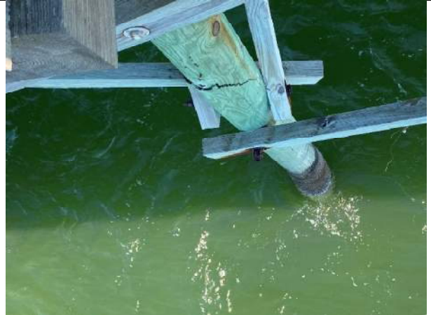
Photo 46: Cracked Pile near station 7+00
