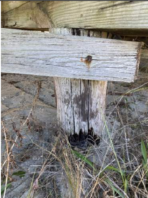
Photo 57: Typical Pile Exterior Rot Deterioration near station 0+00
