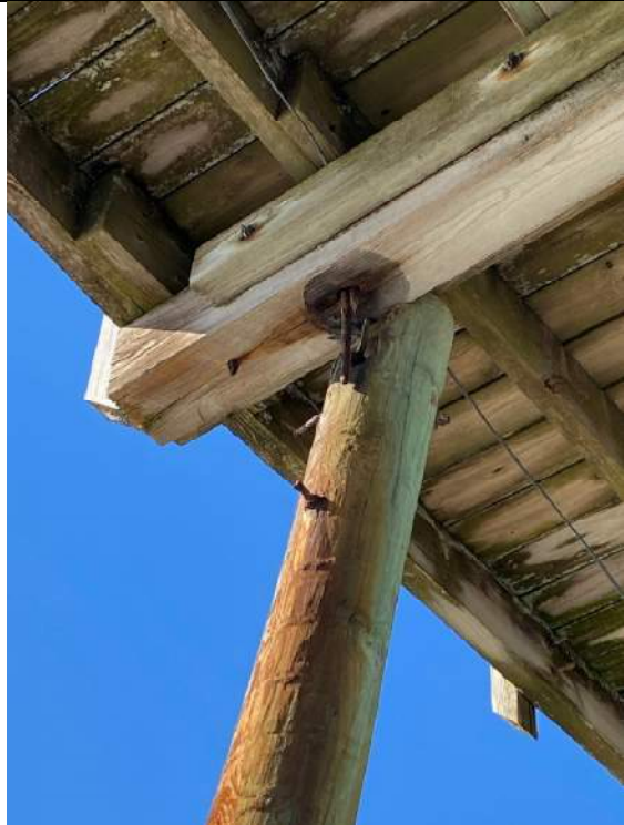
Photo 82: Misaligned Pile Missing Pile / Pile Cap Connection and Missing Bracing near station 3+75
