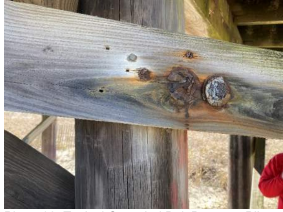
Photo 62: Typical Corroded Bolt Between Pile and Bracing Member near station 0+75
