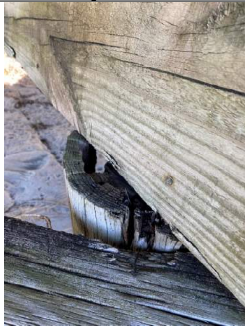
Photo 58: Typical Hollow Pile Deterioration near station 0+00
