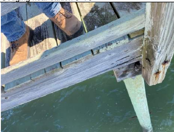
Photo 23: Corroded Connection and Checking at Rail Post and Timber Pile Cap Beam. Pile with Missing Brace and near station 4+00
