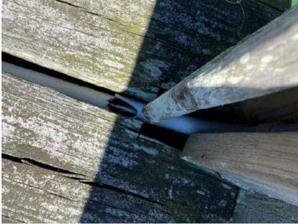
Photo 31: Typical Conduit Housing Damage near station 4+75
