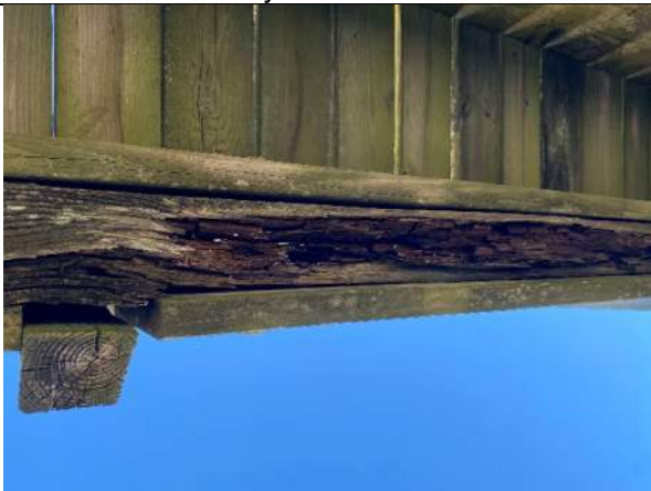
Photo 65: Typical Rotting Joist near station 0+90 Balcony
