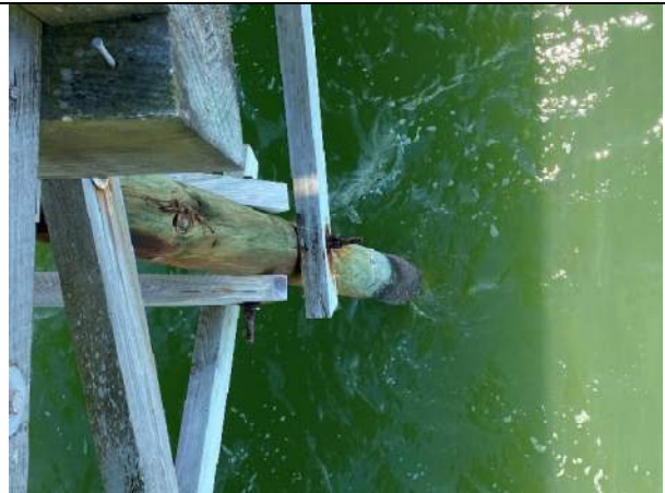
Photo 34: Typical Corroded Bracing Connection Bolts with Pile Gouging near station 5+50
