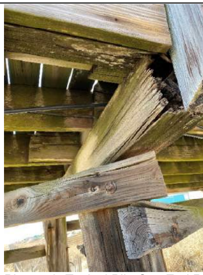
Photo 72: Typical Pile Cap End Rot near station 1+50
