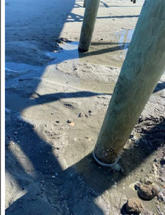
Photo 77: Typical Pile Marine Growth and Localized Scour in the Tidal Zone near station 2+75
