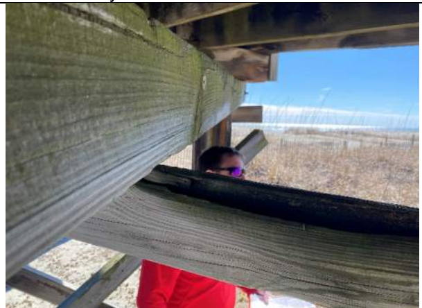
Photo 66: Typical Rotting / Hollow Bracing Member near station 0+90 Balcony
