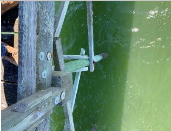
Photo 33: Typical Corroded Bracing Connection Bolts near station 5+00
