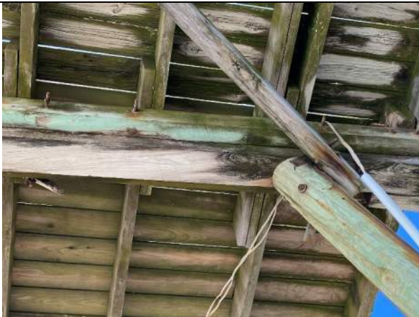
Photo 87: Pile Cap Splicing / Repair near station 4+00
