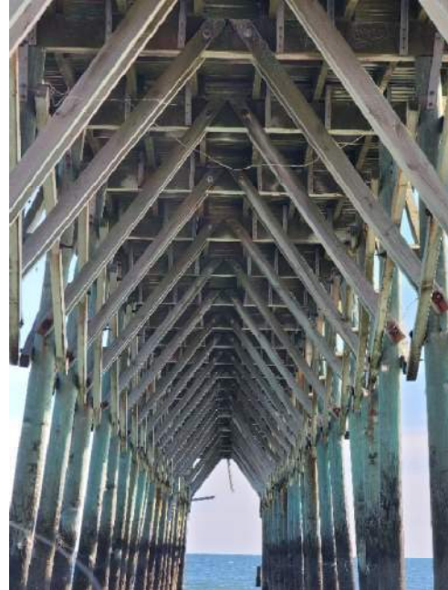
Photo 90: Broken Bracing and Corroded Connection Bolts Beyond station 4+00
