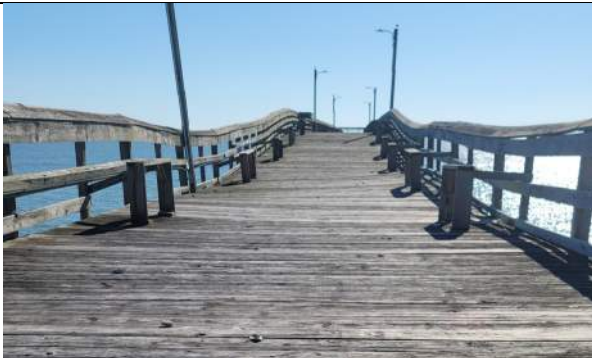
Photo 17: Typical Deck Warping between station 3+25 and station 4+10
