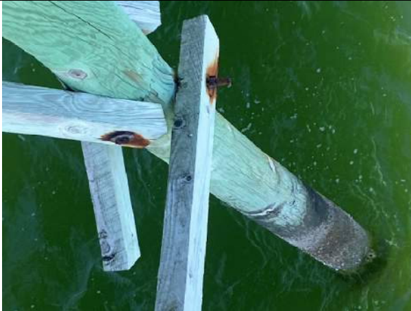
Photo 51: Typical Pile Gouging and Checking near station 7+25
