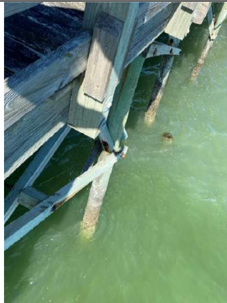
Photo 30: Typical Corroded Bracing and Pile Connection near station 4+25
