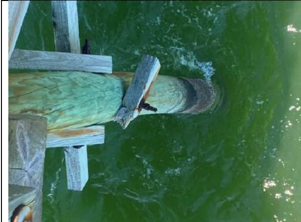
Photo 49: Typical Broken Bracing Member and Corroded Bolts near station 7+25
