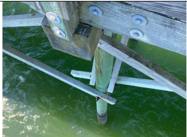
Photo 40: Pile Checking and Gouging near station 6+50
