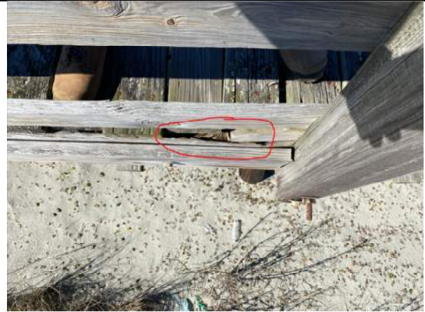
Photo 8: Typical Joist Deterioration near station 1+25
