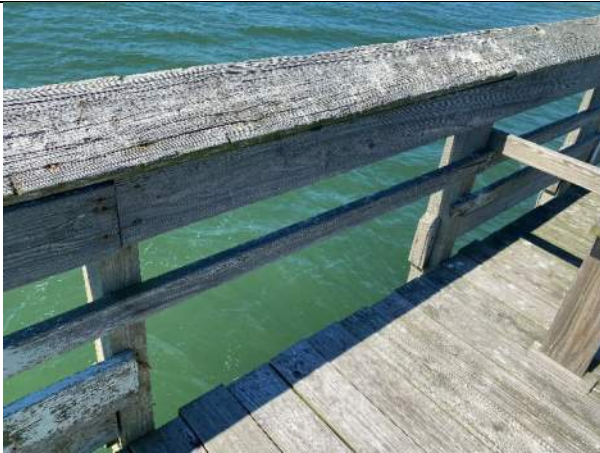
Photo 53: Typical Missing Midrail and Toe Board near station 7+50
