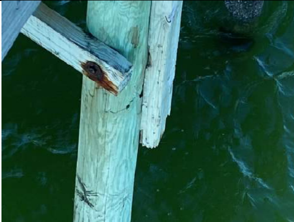
Photo 55: Typical Pile Gouging and Flaking near station 7+50
