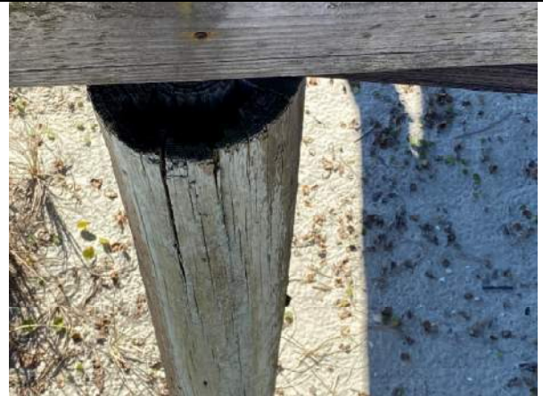
Photo 4: Typical Hollow Pile near station 0+90
