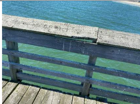
Photo 42: Typical Top Rail Disconnection near station 6+75
