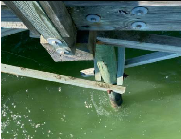
Photo 27: Typical Corroded Bracing Connection near station 4+25
