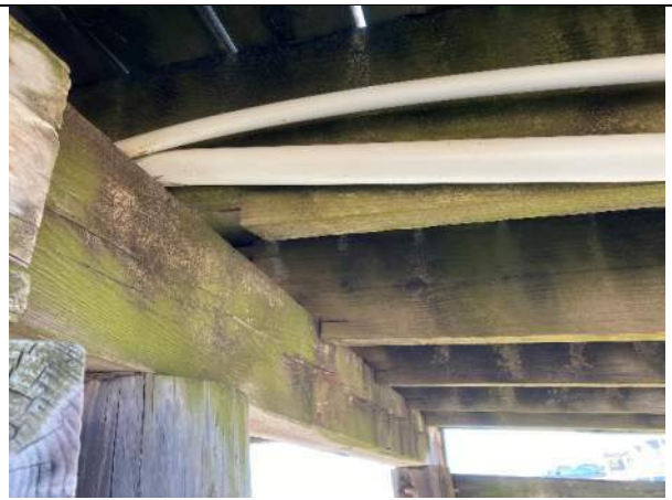
Photo 60: Typical Joist Notching at Support near station 0+75
