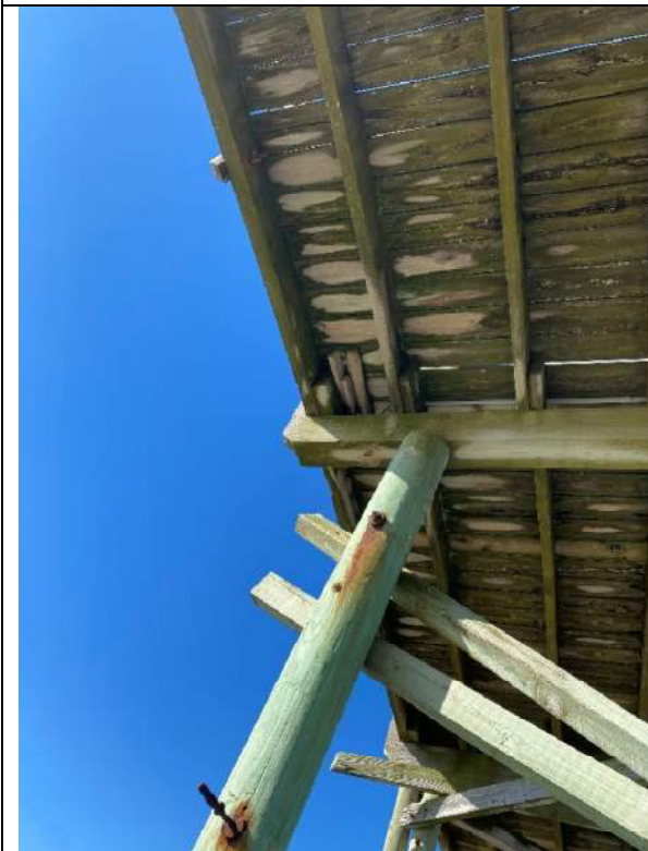
Photo 79: Typical Pile with Missing Cross Bracing and Missing Pile / Pile Cap Connection near station 3+00
