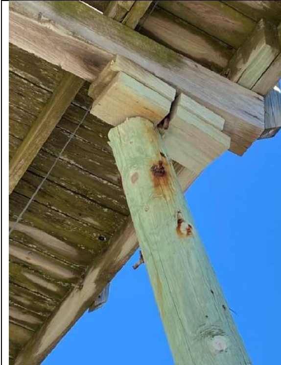
Photo 81: Misaligned Pile Missing Pile / Pile Cap Connection and Missing Bracing near station 3+75
