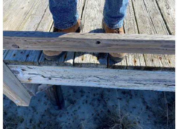
Photo 2: Typical Checking and Flaking at Joists near station 0+90
