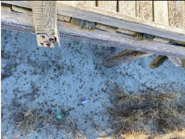
Photo 3: Typical Rail Post Connection Corrosion and Splitting near station 0+90
