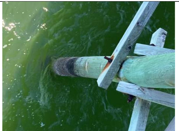
Photo 48: Typical Checking in Bracing near station 7+00
