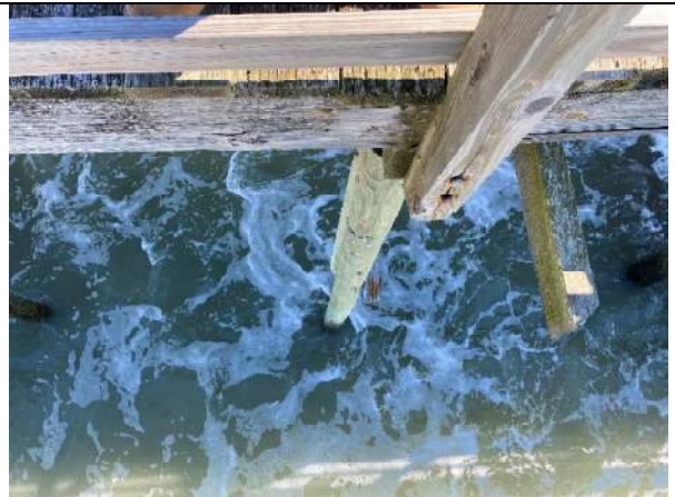
Photo 16: Typical Spliced Pile Repair. Pile with Observed Gouging near station 3+25
