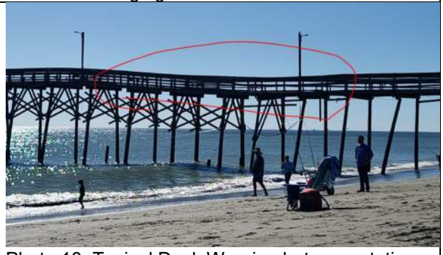
Photo 18: Typical Deck Warping between station 3+25 and station 4+10
