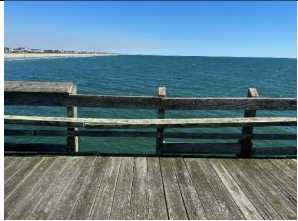
Photo 50: Typical Missing Top Rail and Toe Boards near station 7+25
