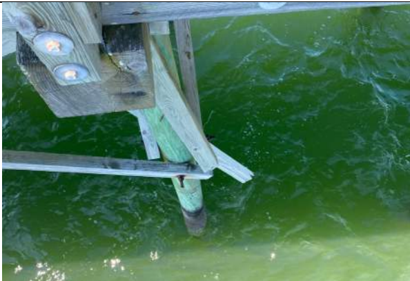
Photo 41: Typical Broken Bracing Member and Pile Cap Checking near station 6+75
