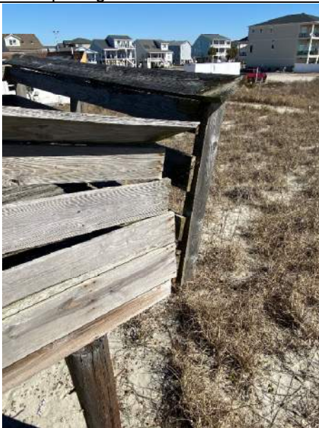
Photo 5: Typical Railing Detachment and Failure near station 0+90
