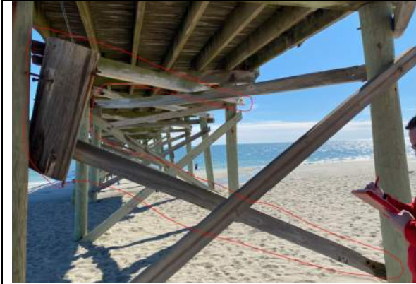
Photo 73: Disconnected Cross Bracing near station 2+25
