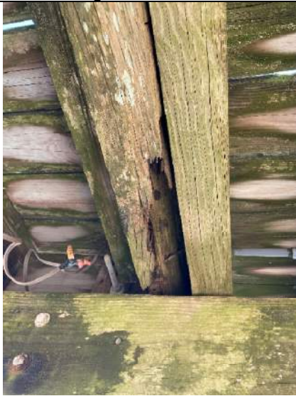
Photo 63: Typical Rotting Joist / Supports near station 0+90 Balcony
