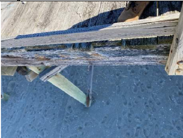
Photo 15: Typical Joist Checking near station 3+00
