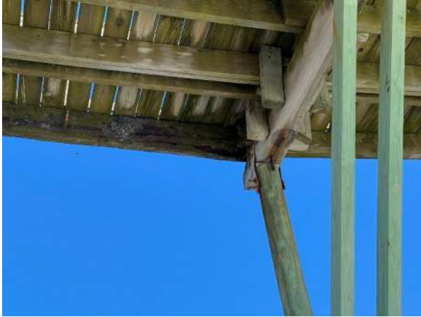
Photo 85: Typical Rotting Joist near station 4+00
