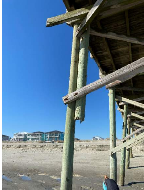
Photo 78: Typical Pile Sistering Repair near station 2+75
