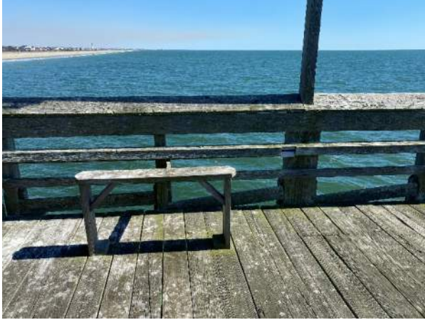
Photo 43: Typical Bench and Disconnected Toe Boards near station 6+75
