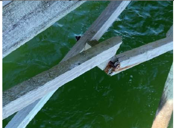
Photo 36: Typical Broken (Disconnected) Bracing near station 6+00
