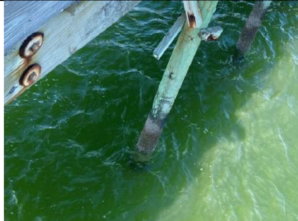
Photo 56: Typical Pile Gouging and Pitting with Broken Bracing near station 7+50
