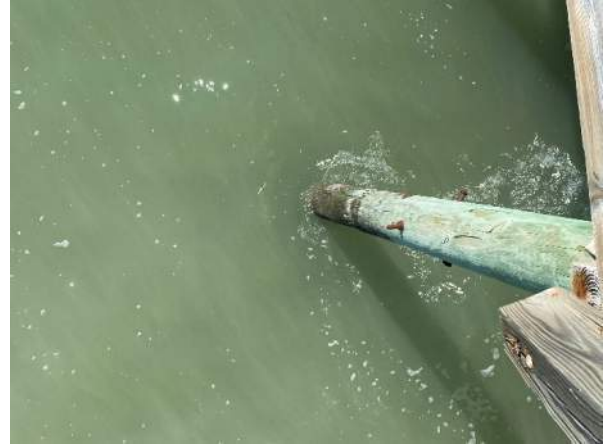
Photo 20: Typical Corroded Pile Bracing Connection with Missing Brace near station 3+75
