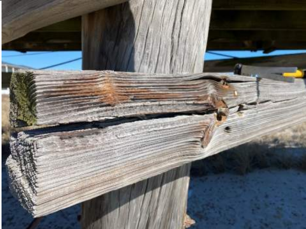
Photo 69: Cross Bracing Checking and Splitting near station 1+00
