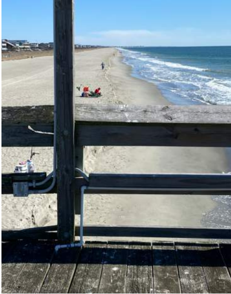
Photo 13: Top Rail Split and Conduit Running along Midrails near station 2+75
