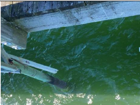
Photo 39: Typical Broken Bracing Member near station 6+50
