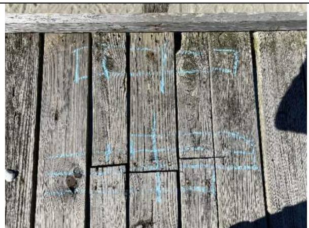
Photo 12: Typical Joist Replacement near station 2+25
