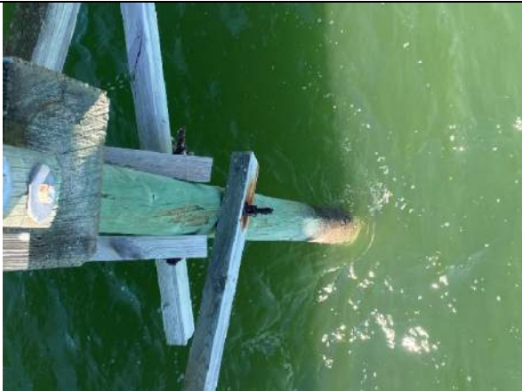
Photo 35: Typical Pile Flaking and Gouging near station 5+75
