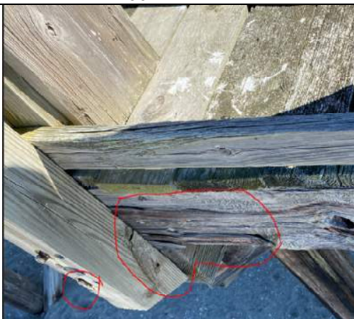
Photo 11: Typical Joist Checking Along Joist and Corroded Connection Bolt near station 2+00
