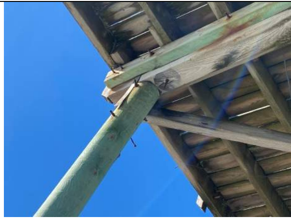
Photo 88: Disconnected Pile / Pile Cap Connection and Corroded Bolts near station 4+00
