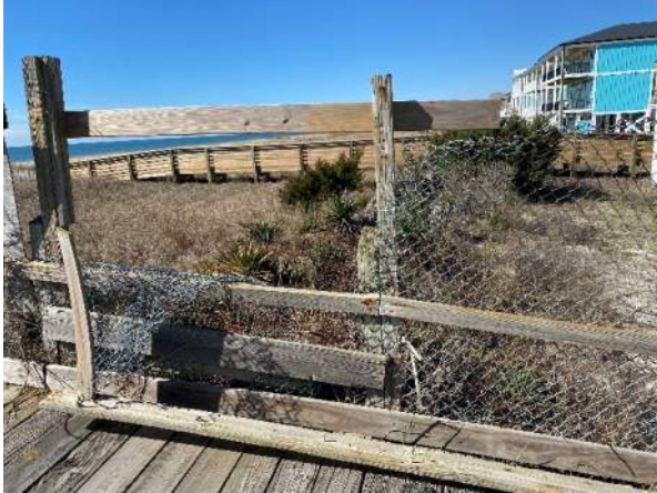
Photo 1: Typical Railing and Fence Damage near station 0+10
