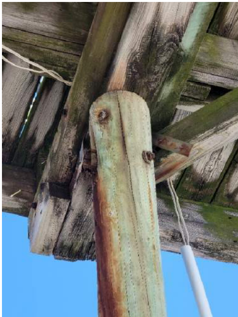
Photo 89: Pile / Pile Cap Connection Failure and Gouging at Pile Top near station 4+00
