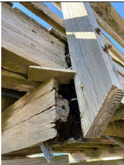
Photo 71: Typical Pile Cap End Rot and Detached Railing Post near station 1+25
