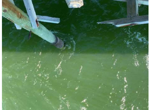
Photo 44: Typical Broken Bracing Member and Corroded Bolts near station 6+75
