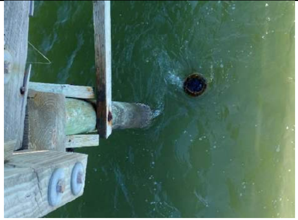
Photo 28: Typical Replacement Pile with Previous Cut-off Pile in Water near station 4+25
