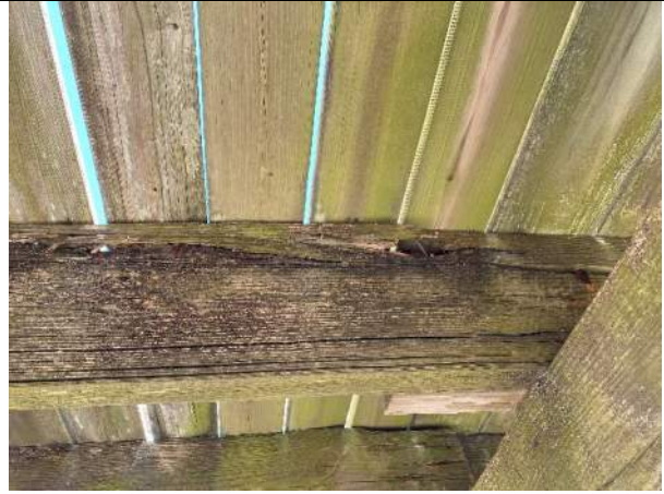
Photo 70: Typical Disconnected and Split Joist near station 1+00
