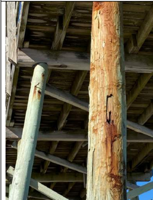
Photo 83: Pile Gouging and Flaking near station 3+75
