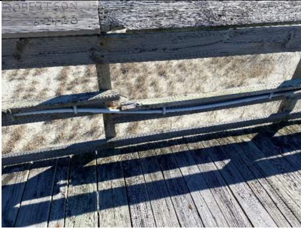
Photo 7: Typical Midrail Separation near station 1+25
