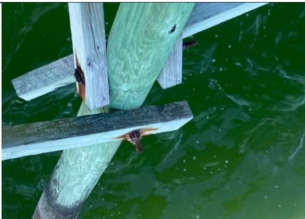
Photo 47: Cracked Pile near station 7+00
