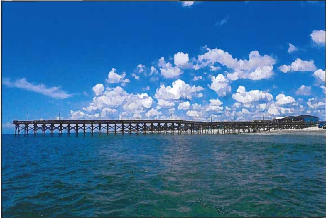
Photograph 1: Overall of Holden Beach Pier.
