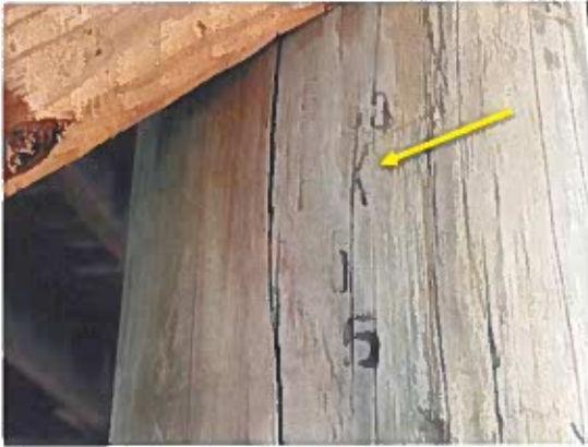
Photo 1 - Brand on pile indicating southern pine and CCA treatment (i.e. "SPSK").
