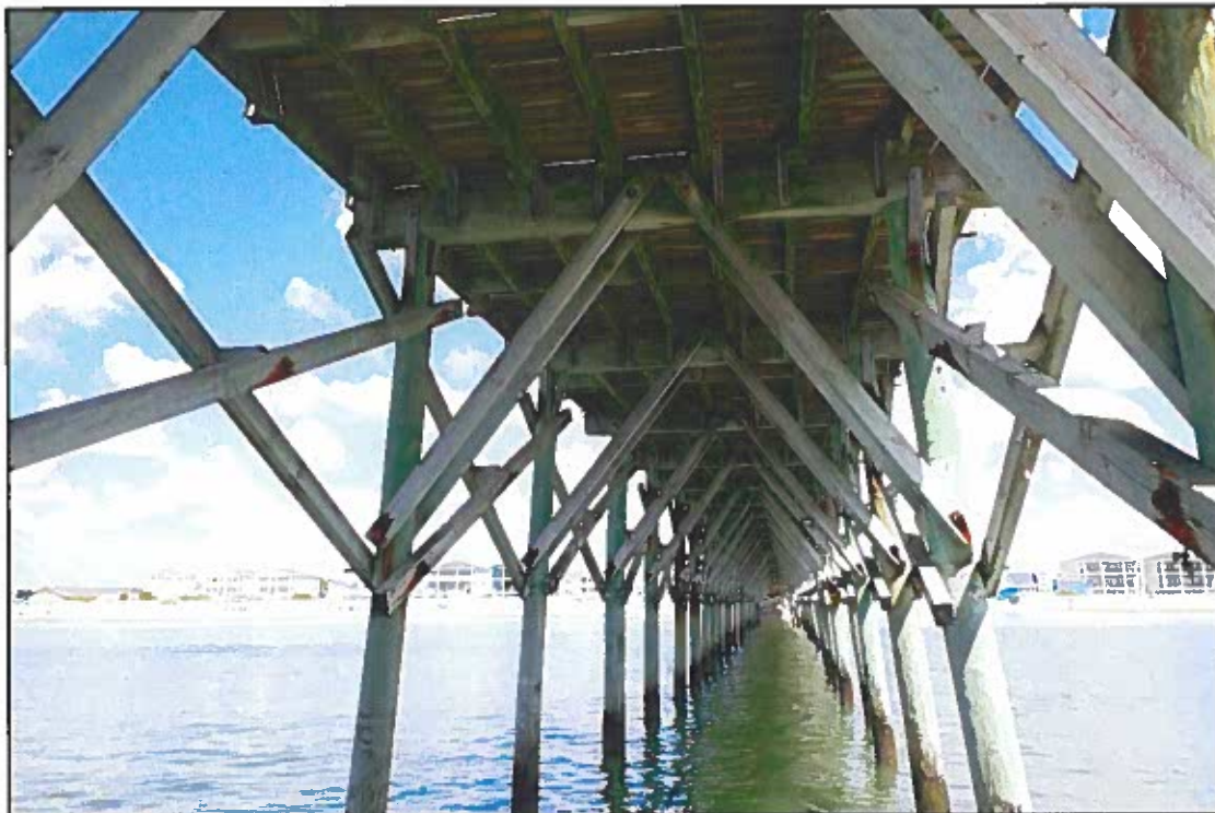
Photograph 2: Typical bent configuration, looking north.
